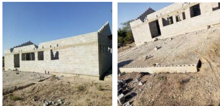
Incomplete Martenity Annex at Nakowa Clinic
