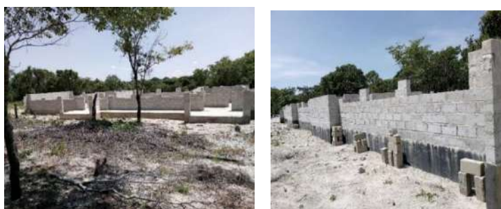
Uncompleted 1x3 Nalinanga Community school
