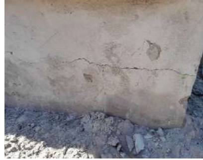
Cracked wall
