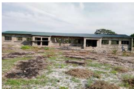
Uncompleted 1x3 CRB at Nakatondo Community School
