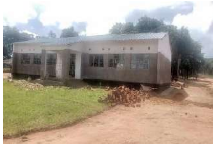
Incomplete classroom block
