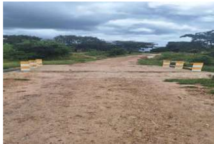
Lusibi bridge measuring 5m wide
