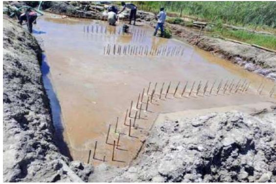
Incomplete Bridge at Chitete stream
