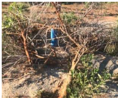
Borehole with installed hand pump and civil work
