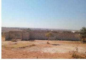
Incomplete Police Post
