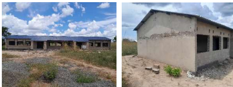
Uncompleted 1x3 CRB at Kaloli Community School
