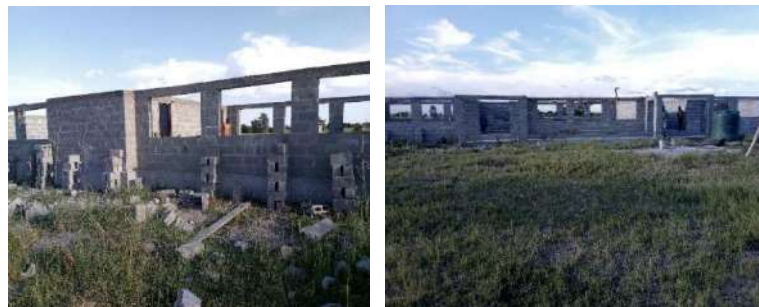
Uncompleted 1x3 CRB at Nalwamba Community School
