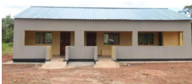
Non-operational but Completed Health Post at Chokwe
