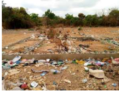
Incomplete Ablution Block Mokambo Market
