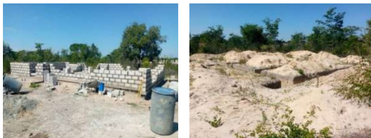
House No. 01 at window level House No. 02 only foundation trenches had been done
