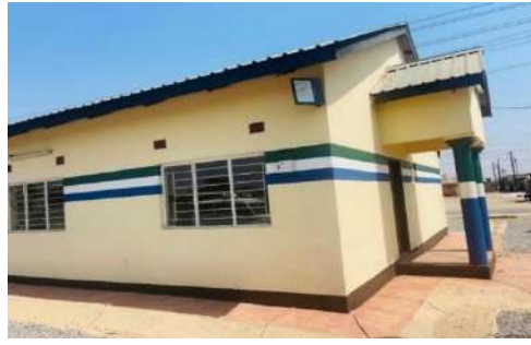
Commissioned police post but not operational-Kamanga
