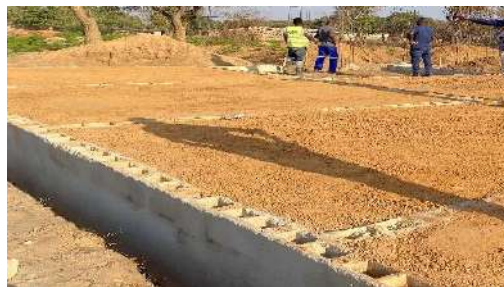
Incomplete Chishikishi Rural Health Centre
