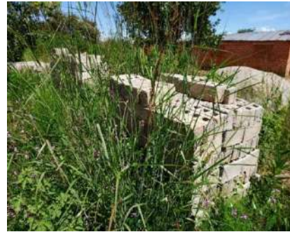
Unused Material on Site
