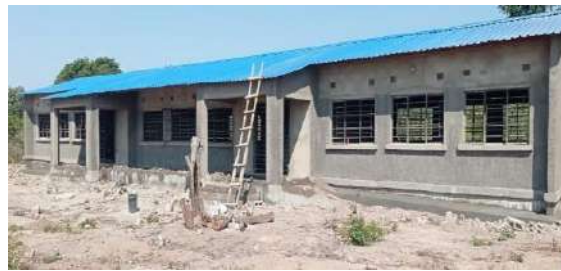
Uncompleted 1x3 CRB at Kafwasonyi Community School
