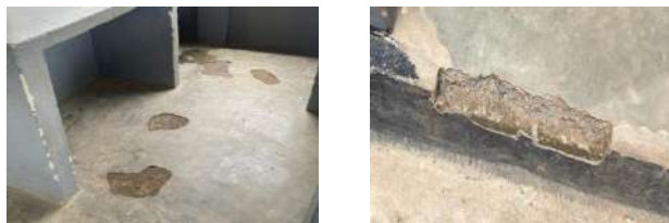
Cracked Floor
