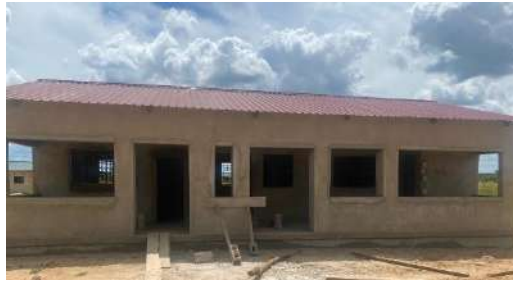
Uncompleted Kaoma-Ndonga Health Post
