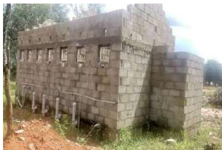
Incomplete water borne toilets
