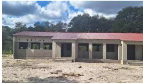
Uncompleted 1X3 CRB at Makwaza Community School
