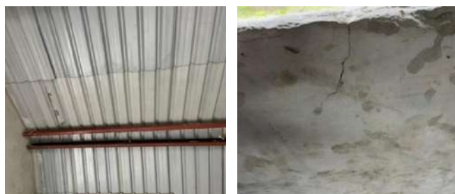
Makwaza Classroom Block
