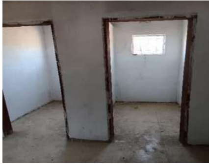
Doors and window not fitted
