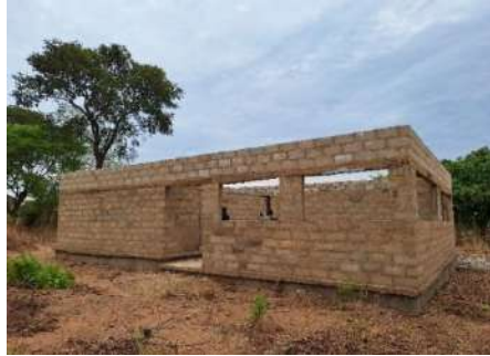
Incomplete Kayisaka Health Post at gable level
