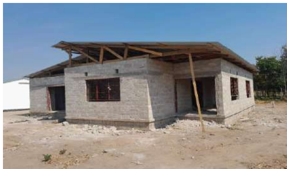
Incomplete theatre block
