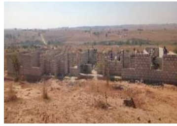
Incomplete semi-detached house
