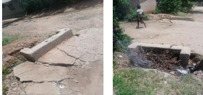
Cracked slab
