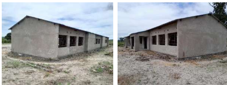
Uncompleted 1x3 CRB at Njatanga Community School
