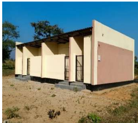
Newly constructed ablution block
