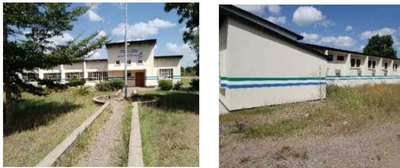
Rehabilitated Police station
