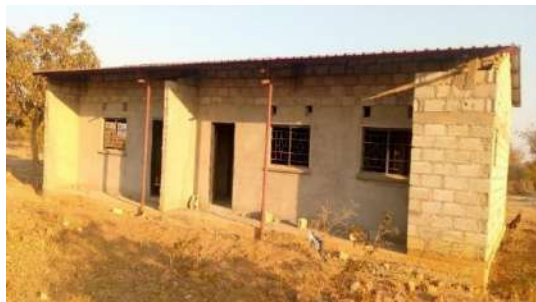
Incomplete Health Post
