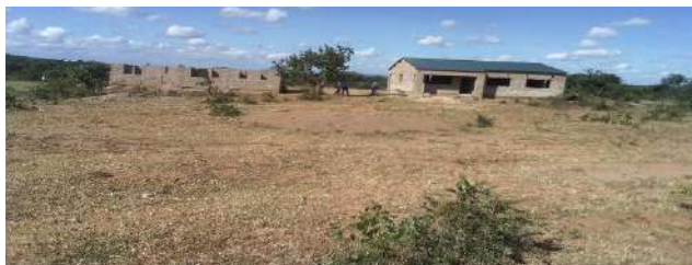
Incomplete Staff Houses at Chibondo
