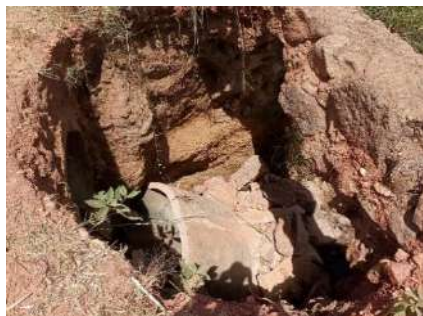
Broken culvert at 8.0 Km
