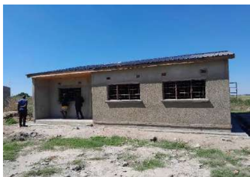
Incomplete staff house
