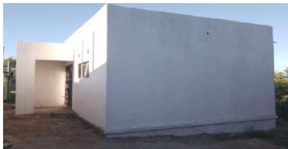
Incomplete Ablution Block at Kariba Secondary School
