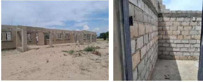
Uncompleted 1*3 CRB at Kaaba Hill Primary School
