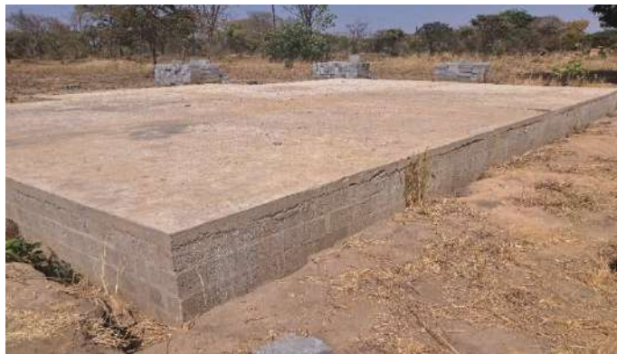
Stalled Police Post at Slab Level
