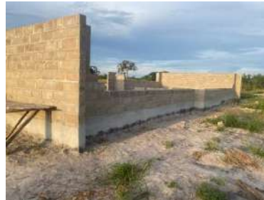
Uncompleted 1x2 CRB at Libinga School
