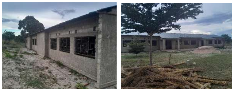
Uncompleted 1x3 CRB at Kashinzi Community School
