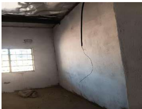
Incomplete Wiring
