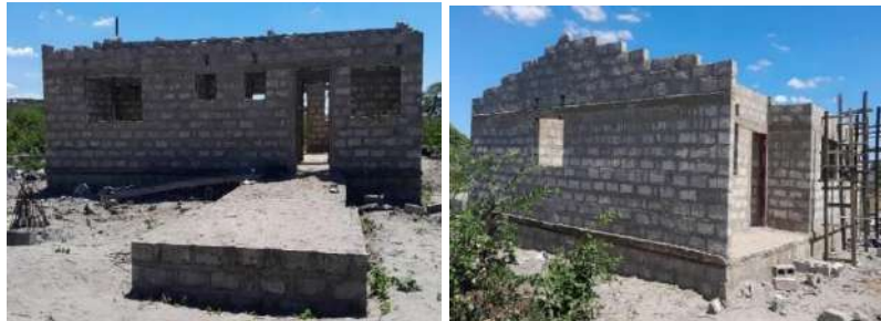
Incomplete staff house
