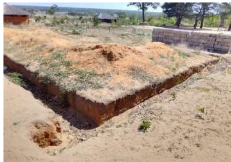
Figure 3-Footing Stage Makumba CRB
