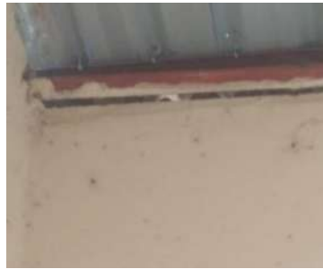
Truss Separated from the Wall
