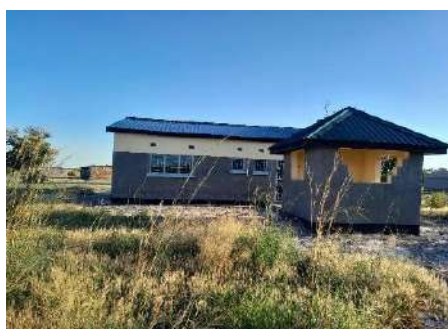
Incomplete staff House and Kitchen
