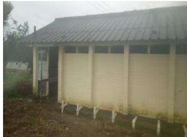
Unpainted ablution block
