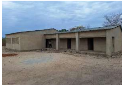
Uncompleted Kanunu Health Post
