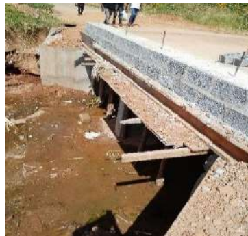
Dambo road Culvert under construction
