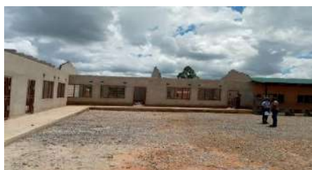
Incomplete 1x5 classroom block at Kamakonde Primary School
