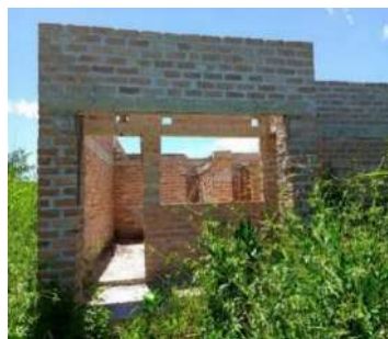
Structure at roof level
