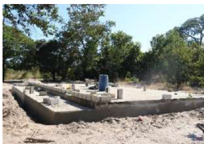
Figure 10 -Slab Level at Nakayembe Maternity Annex
