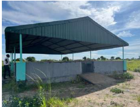
Completed market not in use
