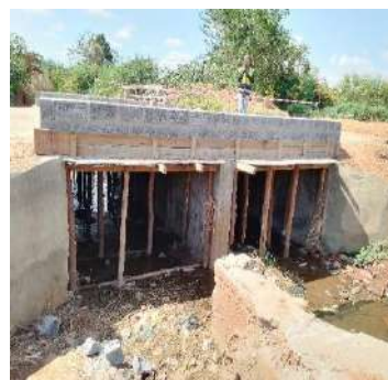
Dambo road Culvert under construction
