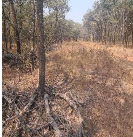
Opening of a Road Without Grading
