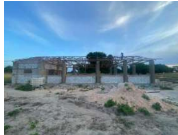
Uncompleted Market Shelter at Longe
