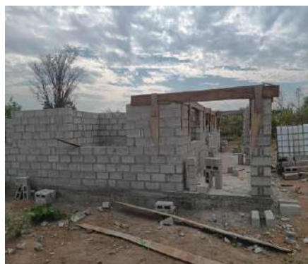
Ring beam being constructed
