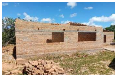
Uncompleted Mulwazi Health Post.
