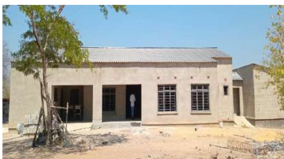
Incomplete Hachibozu Rural Health Post
