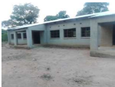
Incomplete classroom block
