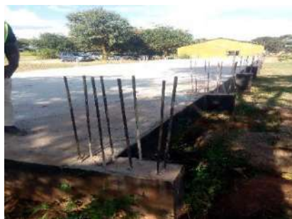
Incomplete 2x3 Storey block
