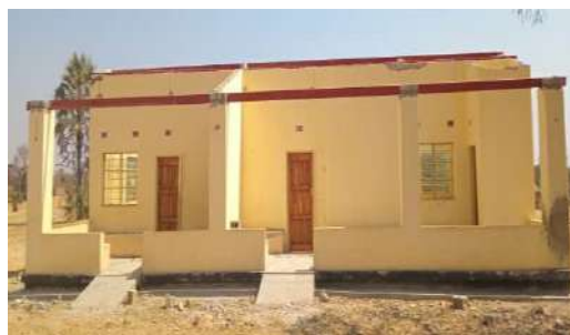
Maternity Wing at Kabanze-Mayobo Rural Health Post
