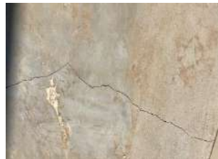
Cracked floor
