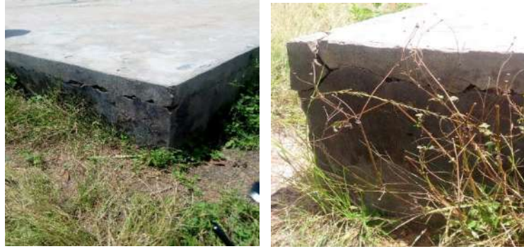
Cracked Slab
