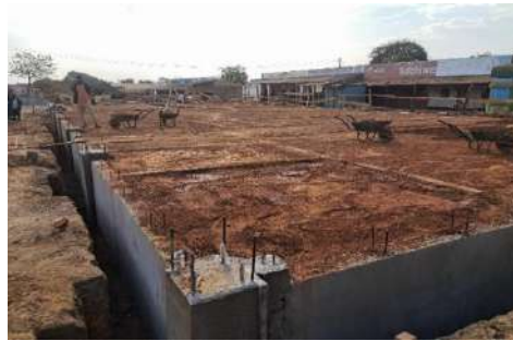
Transit Bus Station at Backfilling Stage
