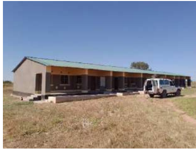
Incomplete Classroom block
