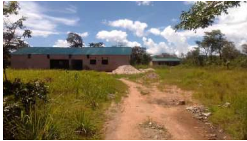
Incomplete health post and staff house
