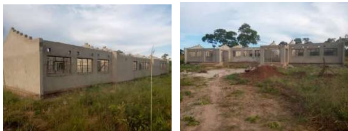
Uncompleted 1 x 3 CRB at Kasheke Community School
