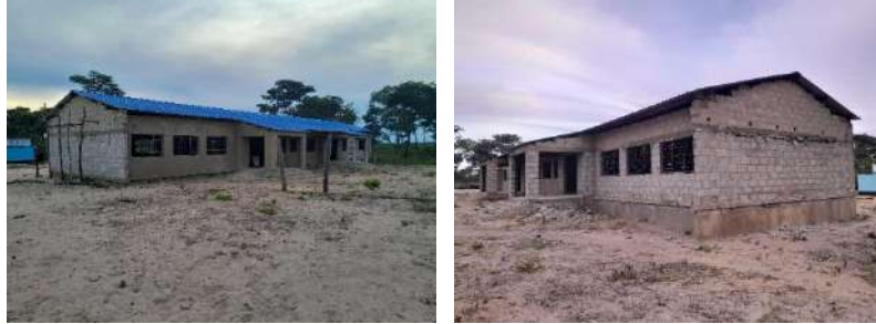
Uncompleted 1x3 CRB at Kachakala Community School
