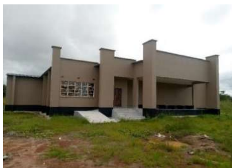
Non-operational but completed mortuary
