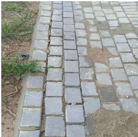
Separating paver bricks
