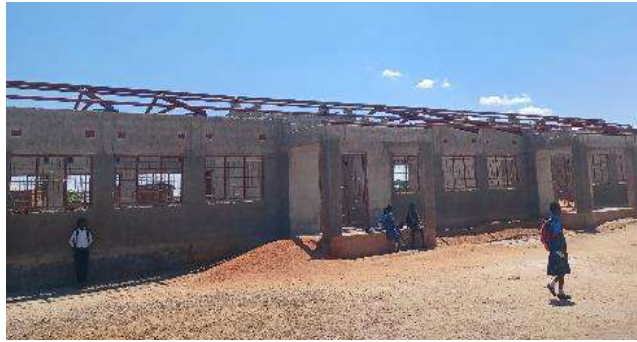
Incomplete 1x3 Classroom Block at Lugwasho
