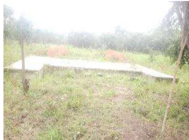
Toilets at slab level
