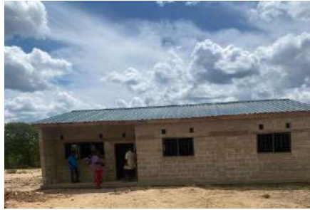
Uncompleted Staff House at Kaoma-Ndonga Health Post
