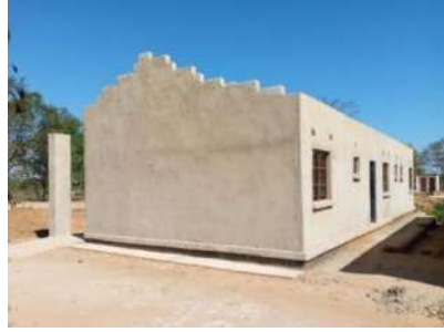
Maternity Annex at Chinkozya Health Centre
