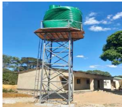
Figure 9 -Side View of Tank Stand and Maternity Annex
