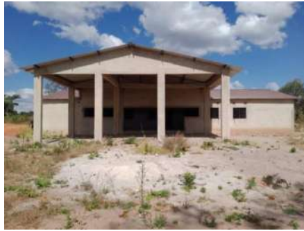
Incomplete Rural Health Post
