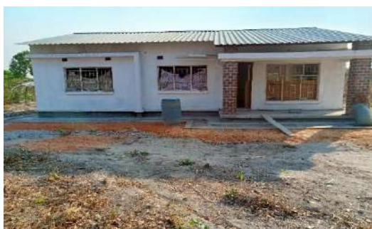
Staff house at Kabangamika Health Post
