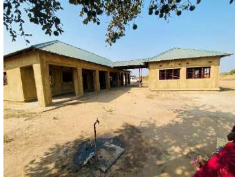
Unpainted Mothers' Shelter without glazing
