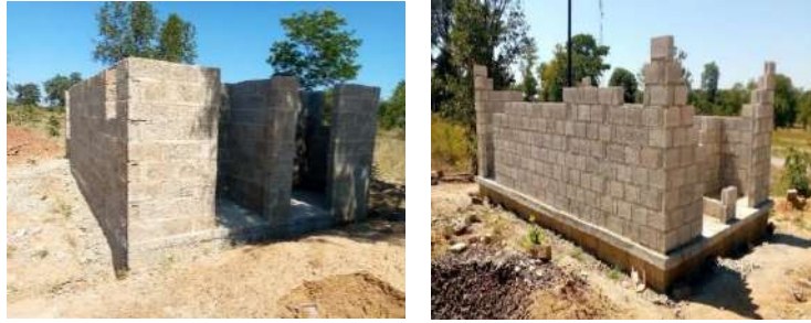
Ablution block 1 and 2 at window level
