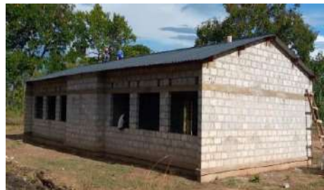
Uncompleted 1x2 CRB at Kajejeje School
