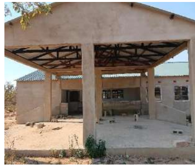
Incomplete floors and ceiling board
