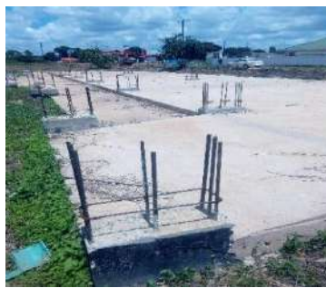
Slab Done at Mushitala Sec School for 2x3 Storey Block
