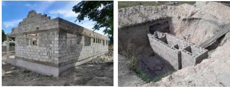
Uncompleted Mothers Shelter at Mangango Hospital
