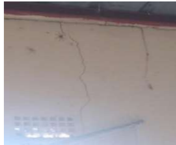
Cracks on the Wall
