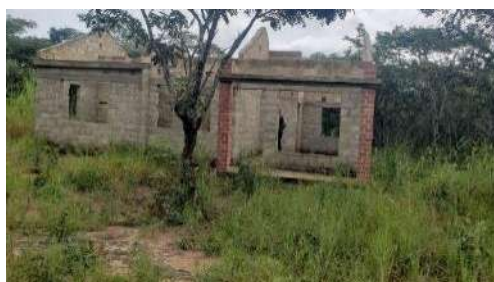
Incomplete staff house
