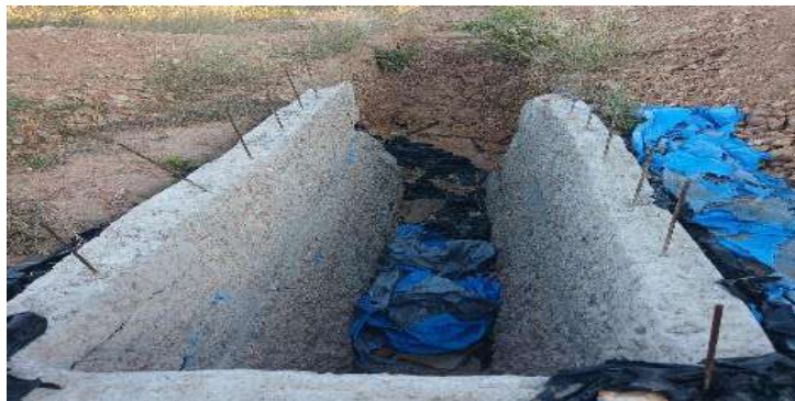
Incomplete Dip Tank in Siatembo
