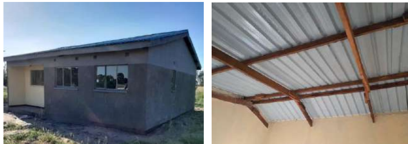
Incomplete staff house
