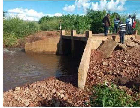
Washed away stone pitching areas of the Constructed Gondar Bridge
