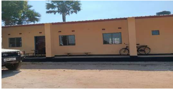
Non-operational but Completed Maternity Annex at Kapesa Rural Health Post
