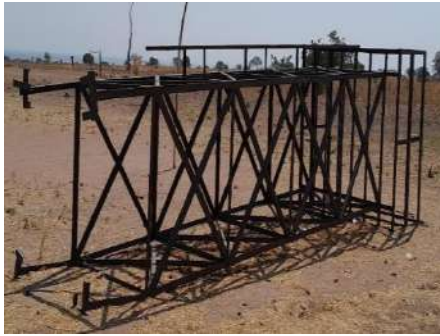
Water tank still not erected
