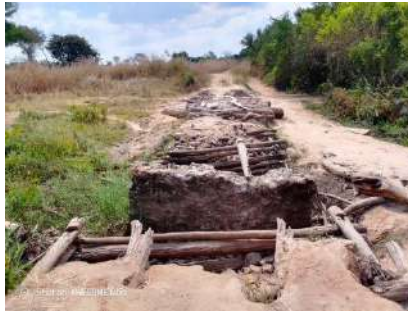
Construction site for Kabisha Bridge
