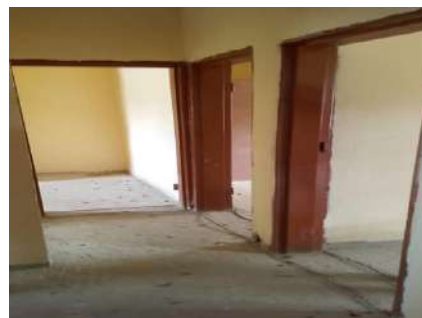
Incomplete staff house
