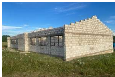
Uncompleted 1x2 CRB at Chilombo School
