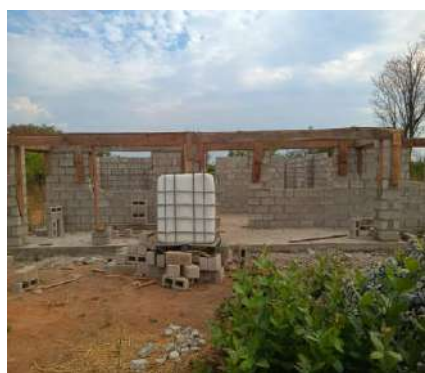
Super structure under construction
