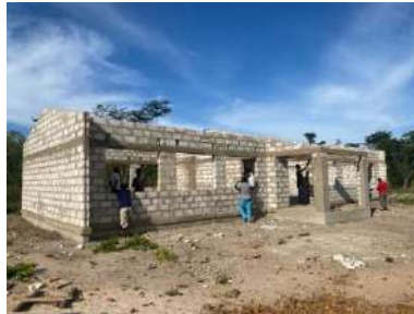
Uncompleted 1x2 CRB at Shitele School
