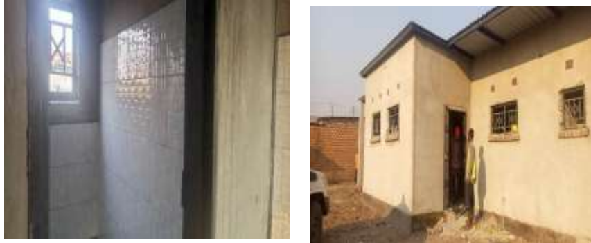
Incomplete Toilet at Chongwe Market
