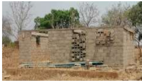
Incomplete Staff House and Guard House
