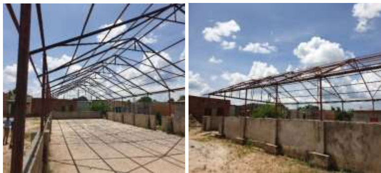
Market shelter under construction
