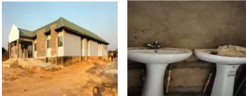
Construction of the Civic Centre
