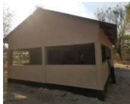
Completed and Non Operational Mini Bar
