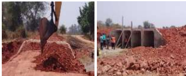
Uncompleted Crossing Point
