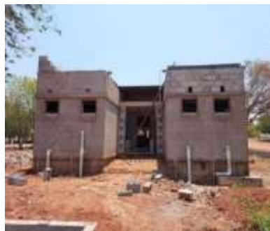
Incomplete Bar and restaurant at Chipepo Guest House
