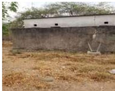
Toilet Structure not in use
