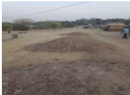
Part of the incomplete 1km stretch
