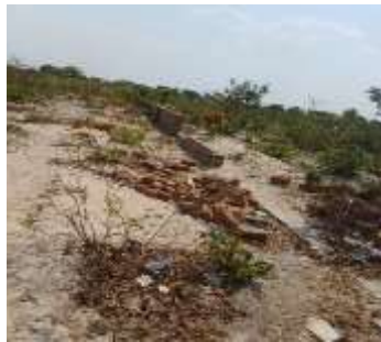
Incomplete Fence at the Dump Site
