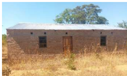
Incomplete staff house - Katanda Ward
