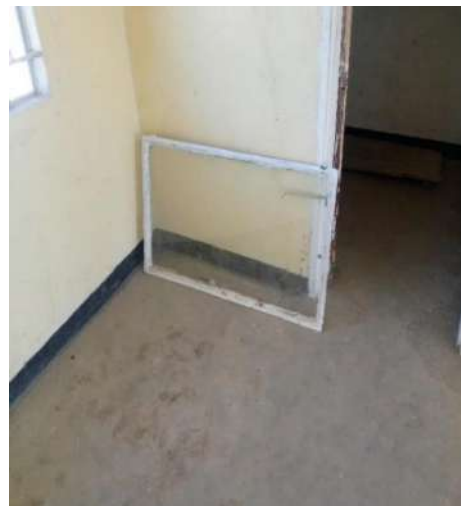
Part of the window has fallen off
