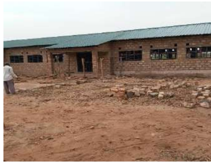
Incomplete 1x3 Classroom Block - Mayenu
