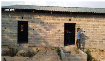
Incomplete Health Centre
