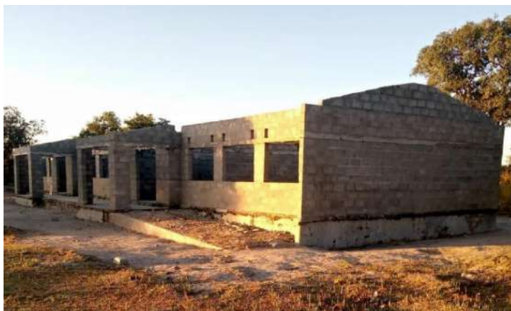
Incomplete 1x3 CRB
