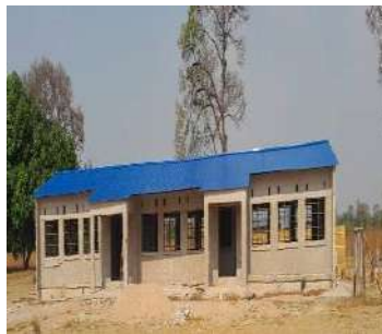
1x3 Classroom Block at Shishamba Primary School
