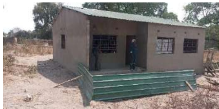
The uncompleted Staff House at Nasilimwe RHC
