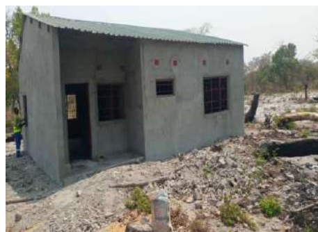
Incomplete staff house
