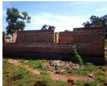
Abandoned Project Kalulu Primary School
