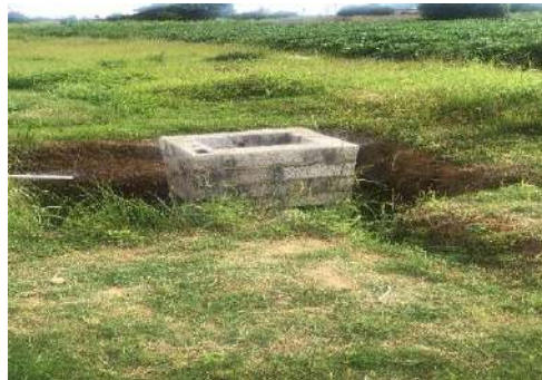
Stalled works construction of -Ablution Block and Soakaway
