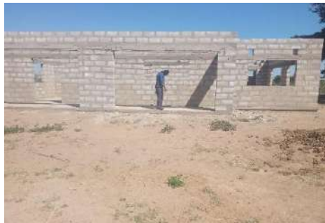
Incomplete maternity annex
