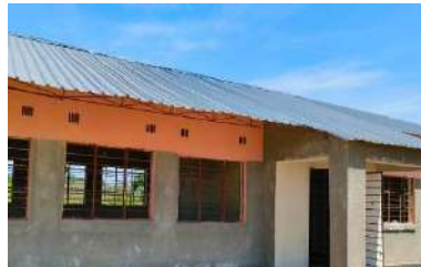
Roof at Chathomba Primary School
