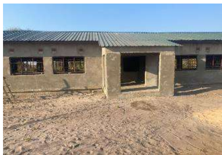
Uncompleted CRB at Nang'oko Multi-Skilled Centre
