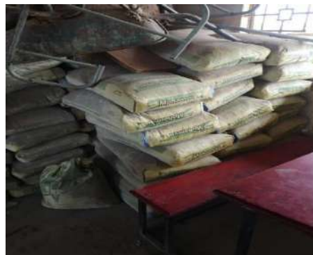
Hardened pockets of cement
