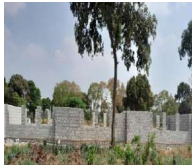
Delayed completion of 1x2 CRB at Mbumisha Community School
