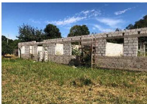
Classroom block under construction
