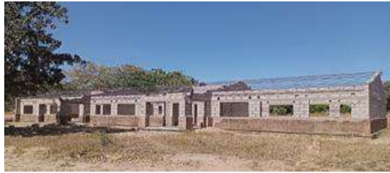
Incomplete 1x3 CRB
