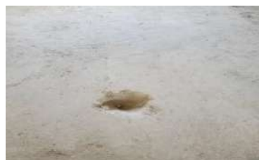
Floor screed removed
