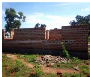
Abandoned Project Kalulu Primary School
