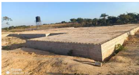
Civic Centre at Slab level
