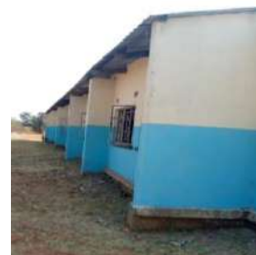
Spoon drain final coat for paint not done
