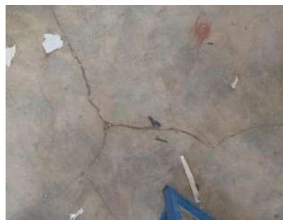
Multiple cracks on the floor in all the three (3) classroom blocks
