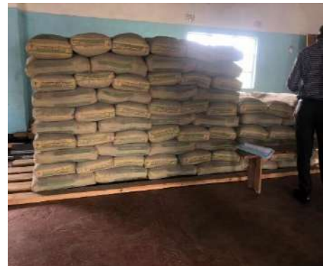
Uncompleted Classroom block and Caked Cement
