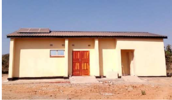
Mortuary at Thendele Level one Hospital
