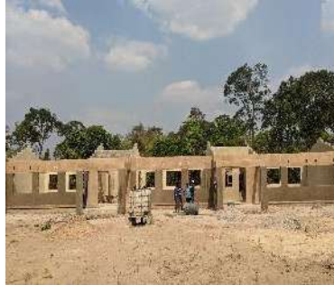
1x3 CRB at super structure
