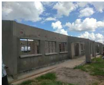
Incomplete 1x3 Classroom block at Gable Level
