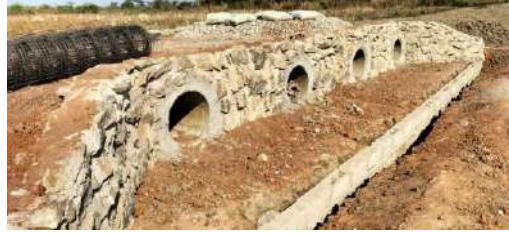
Uncompleted Culvert in Mwalala Ward
