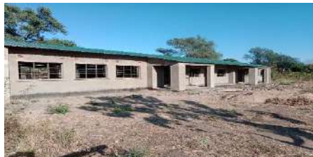
Uncompleted 1x3 Classroom Block
