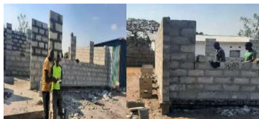
Incomplete 1x3 classroom block
