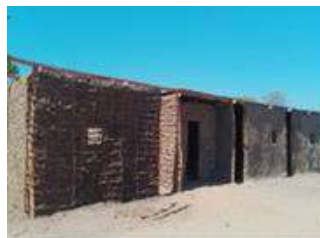
Partly roofed Community School
