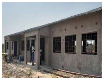
1x3 Classroom Block at Sipalo Primary School
