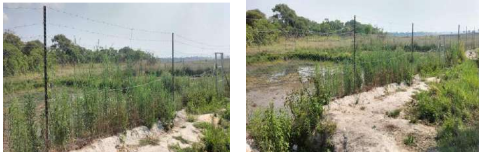
Construction of a Wire Fence
