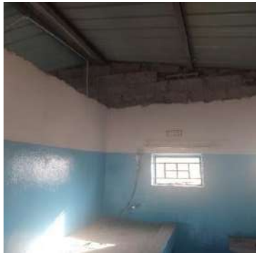
Structure without Ceiling
