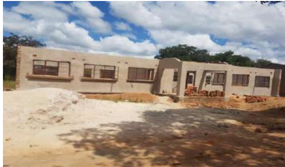
Incomplete 1x2 Classroom block
