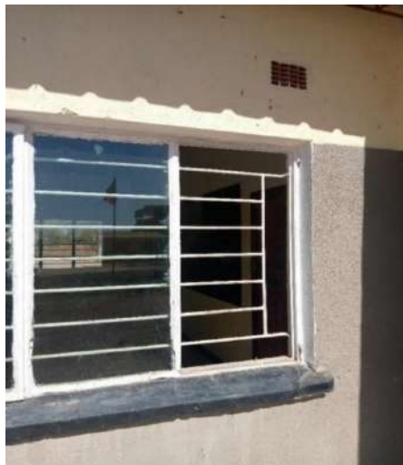
Part of the window has fallen off
