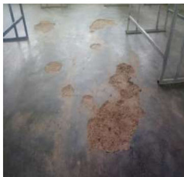
Potholes developed in classroom No. 2 and classroom No. 3
