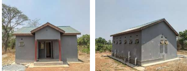
Ablution block at Mushingashi Market without Solar Connection
