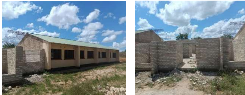
Incomplete 1x4 Classroom Block at Waitwika Secondary School
