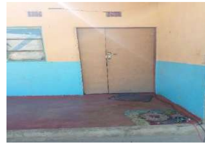
Flush door fitted instead of mukwa
