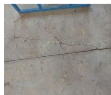
Multiple cracks on the floor in all the three (3) classroom blocks
