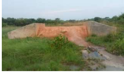
Pipe Culvert on Mwenda - Fisheries Road
