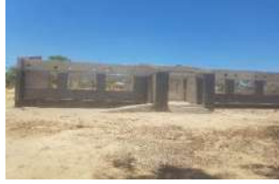
School under construction
