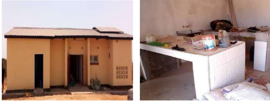
Mortuary not completed at Muyombe Level one Hospital
