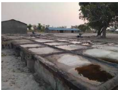
Sisiye CRB at slab level
