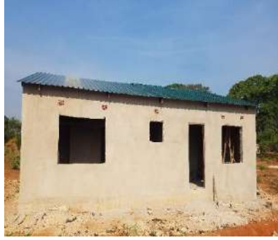
House 1 at roofing stage
