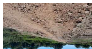
Part of eroded bridge
