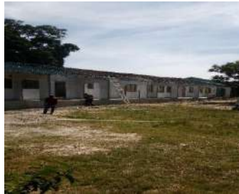
Incomplete IX 3 Classroom block
