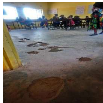
Potholes developed in classroom No. 2 and classroom No. 3
