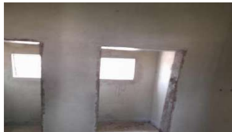
Uncompleted Staff houses at Kalumeyoyo
