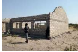
Incomplete 1x3 CRB
