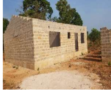
House 2 at gable level
