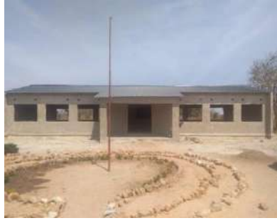
1x2 CRB at Chipandaike under construction
