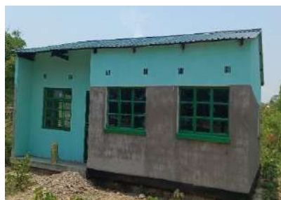
Staff House at Mulanda primary school
