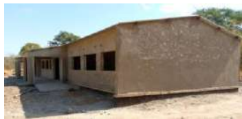
1 x 3 Classroom Block at Kanchele Primary School
