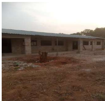
Incomplete 1x3 Classroom Block
