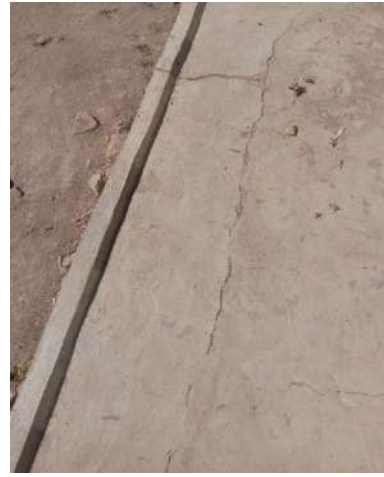
Strong room not fitted with the grill gate Cracks on the spoon drain
