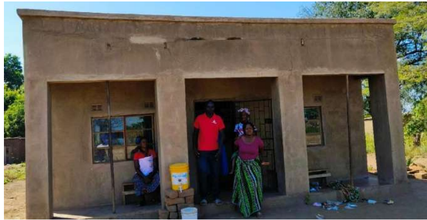
The Shop built by Chipako Women’s Club
