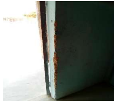
Wall with peeled off plaster
