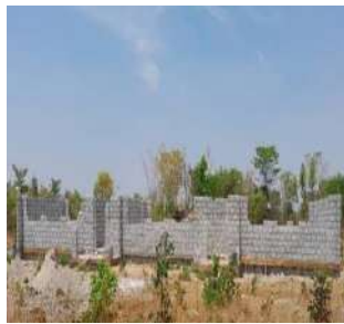
Delayed completion of 1x2 CRB at Kalapu
