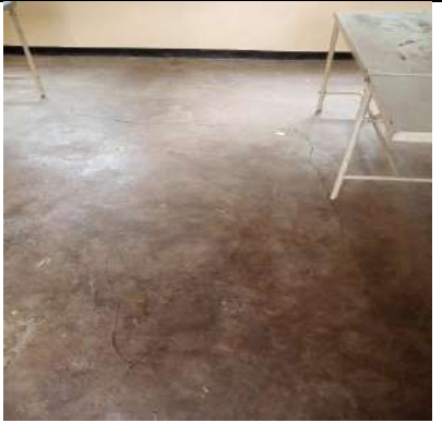
Cracked Floor
