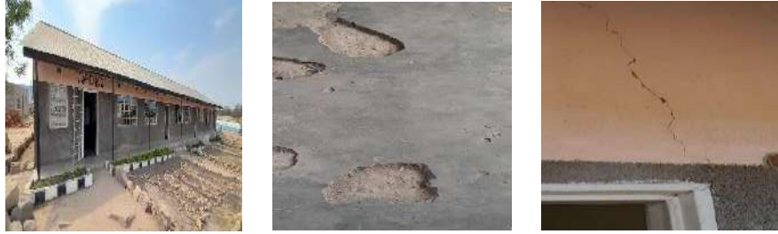
Floor of the classroom block
