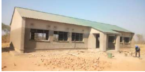
Uncompleted 1x2 Classroom block
