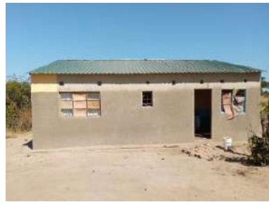
Incomplete staff house at Nachocho Community
