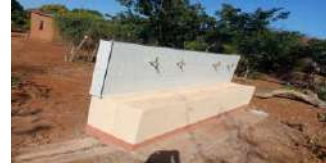
Kiosk without running water
