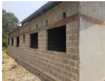
Window frames not done
