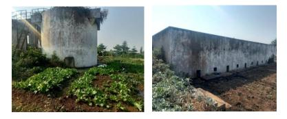
Dilapidated Sediment Tanks with Non-Functional Filters
