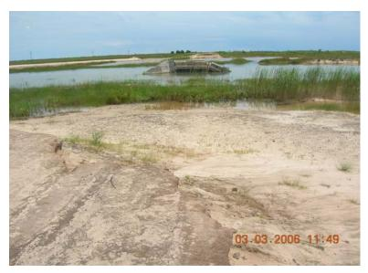
A culvert on a portion of road which was washed away seen as an island
