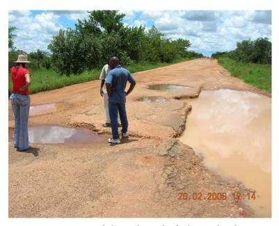
LOT 2- Some parts of the road completely damaged and cannot Support any layer of Tarmac.
