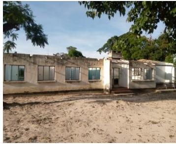
Dilapidated FTI – Sesheke
