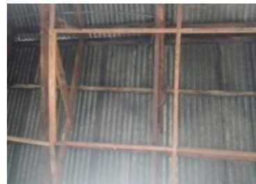
Cell Ceiling without wire mesh
