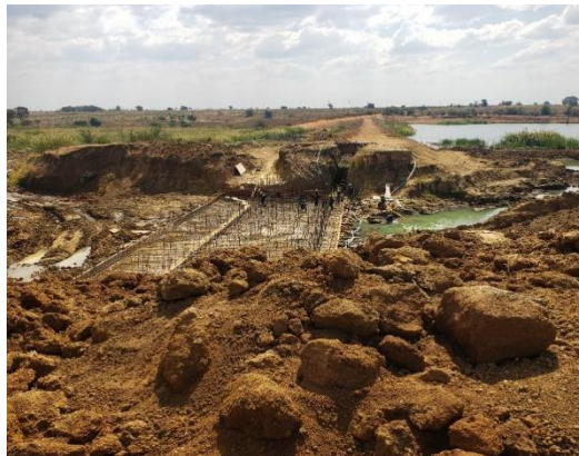
Incomplete Mwase Dam
