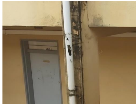
Figure 6.2: Broken gutter pipe and falling off gutters
