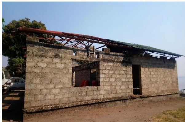
Figure 4.4: Partially roofed kitchen and dining block
