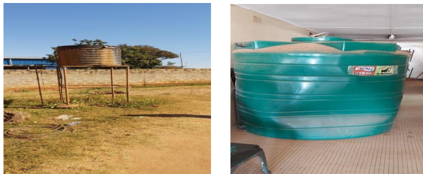
Figure 13.7: Old tank stand and un-mounted new tank
