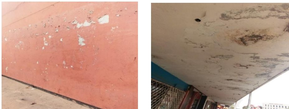
Figure 25.5: Poor painting of Sanlam Building and Leaking Roof – Ex Legal Building in Kitwe
