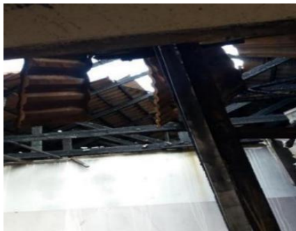
Figure 8.1: Parts of the Walls and Roof Gutted by Fire
