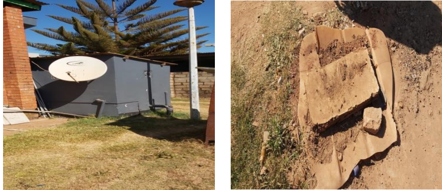
Figure 13.6: Make shift toilet and no manhole covers
