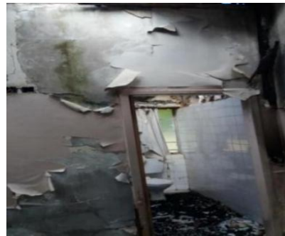
Figure 8.1: Parts of the Walls and Roof Gutted by Fire
