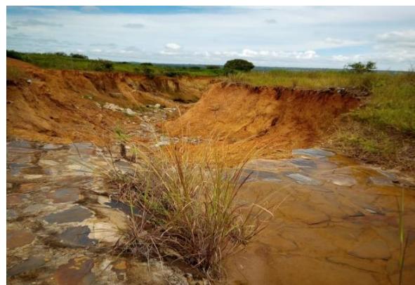
Figure 19.1 : Gulley without Gabion Walls
