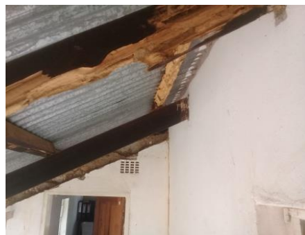
Figure 8.5: Cracked Walls and Damaged Roof Timber
