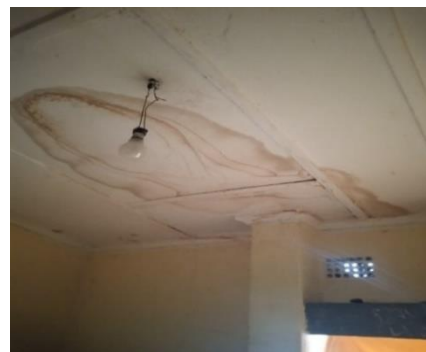
Figure 9.2: One of the Unrehabilitated Houses and Water Marks on Ceiling of a House
