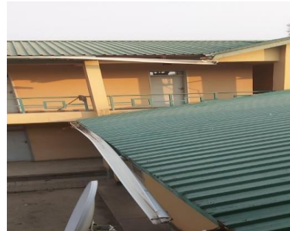
Figure 6.2: Broken gutter pipe and falling off gutters
