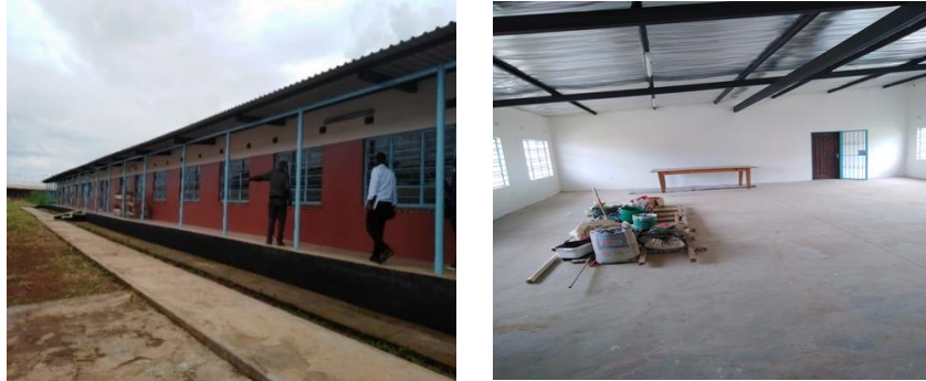
Figure 14.1: Completed building and untiled computer room
