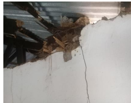
Figure 8.5: Cracked Walls and Damaged Roof Timber
