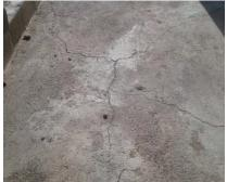
Incomplete Provincial Local Court Office Block with Cracks on the Slab
