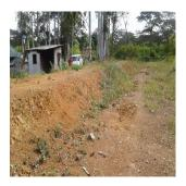
Unrepaired Collapsed Embankment at River Water Pump Station in Mufulira
