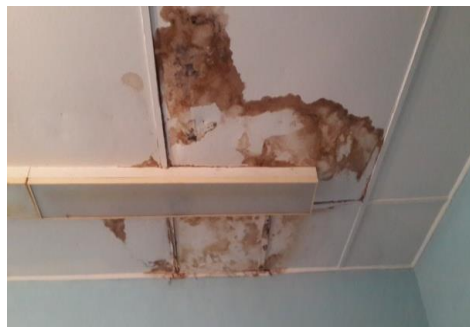
Leaking roof
