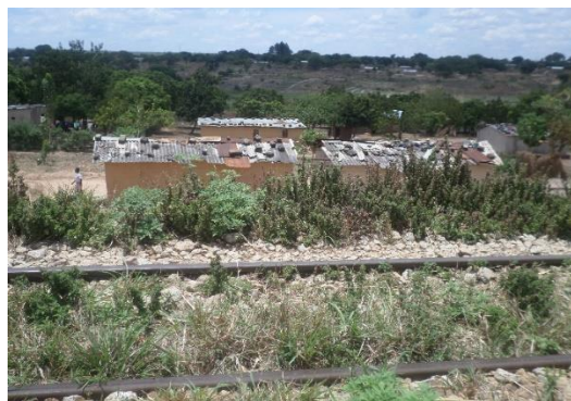
Railway encroachment at Mpika Station
