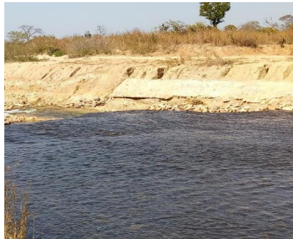
The wall of the embankment
