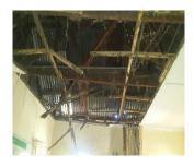
Collapsed ceiling board
