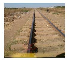
Section between Lusaka and Kafue lacking ballast
