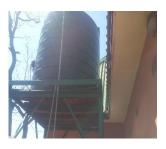
Water tank erected too close to Ablution Bloc
