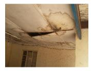
Rotting ceiling board due to leaking roof
