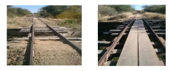
Culverts with inadequate and misaligned sleepers – Mulobezi line
