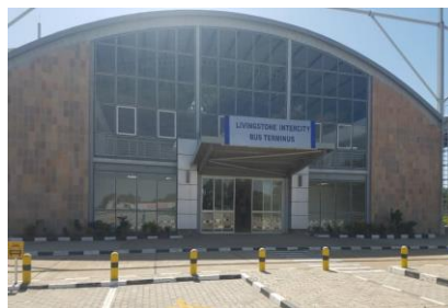
Livingstone Bus Terminus Main Building
