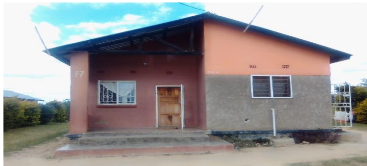
One of the Houses from the Housing Complex in Chibombo
