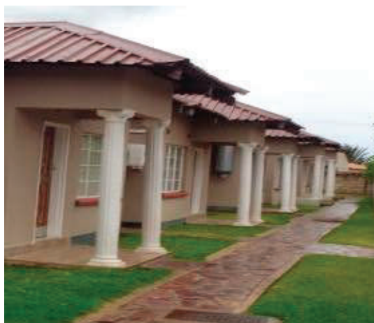
Picture 4.5: Completed Newly Constructed Rooms at Henry Courtyard Lodge
