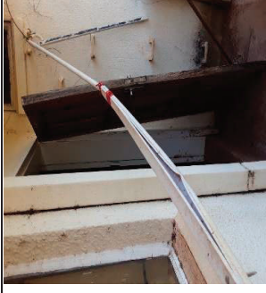
Sign of leakages in the roof Door & Internet Cable not Properly Fixed
