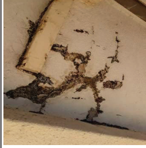
Sign of leakages in the roof Door & Internet Cable not Properly Fixed
