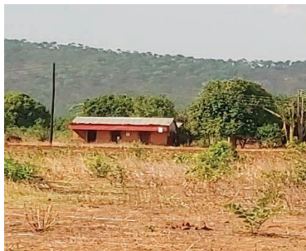
Pictures 18.3: House on encroached Corporation land
