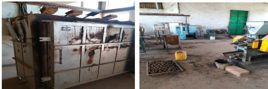
Pictures 10.2: Poorly Maintained Coal Briquette Plant
