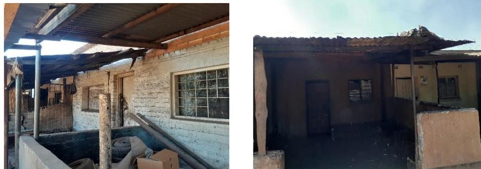
Rotten Roofing Sheets, Broken doors and broken windows
