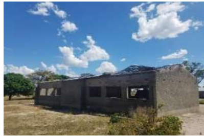
Incomplete 1x2 CRB at Lushushwa Primary School
