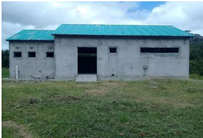
Abattoir under construction
