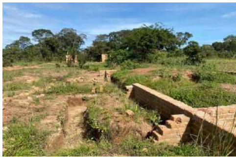
Classroom at Box level at Yamwela Primary School
