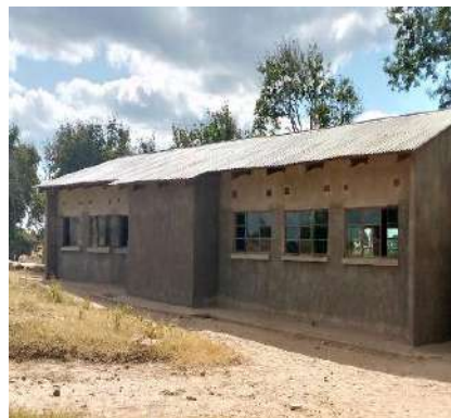
Incomplete 1x2 Classroom Block at Naluama Primary School
