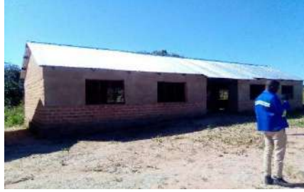
Incomplete Classroom Block at Chifungo Community School
