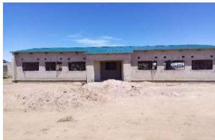
Incomplete classroom block
