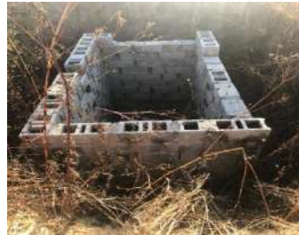
Incomplete Double VIP toilet
