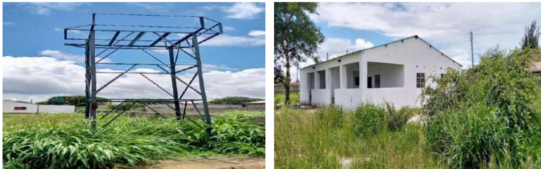
Incomplete installation of water reticulation system in Libala Ward
