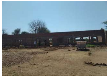
Incomplete 1x3 Classroom Block at Sianyuka Primary School
