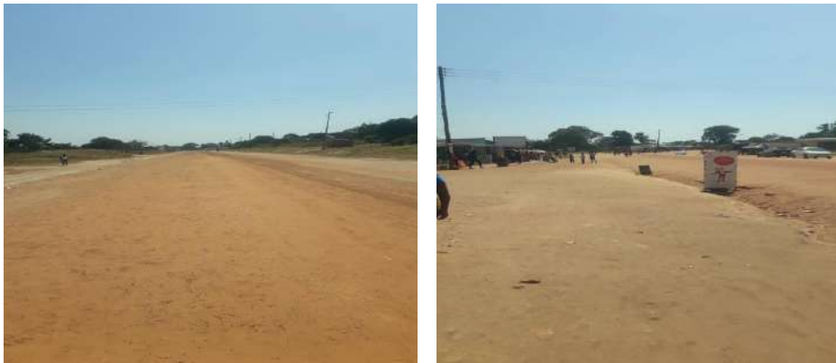
Streets with No street lighting
