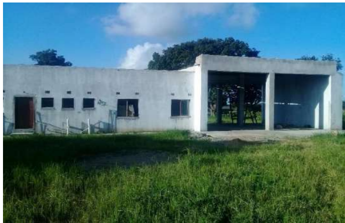
Fire Station under construction
