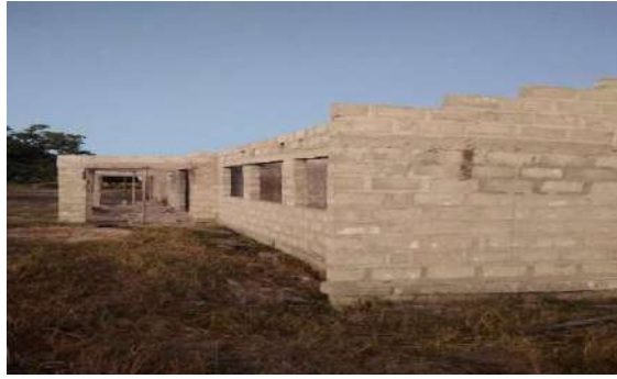
Incomplete 1x3 CRB at Mbaao
