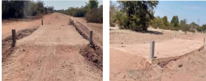
Drift Bridge without levelled concrete approaches
