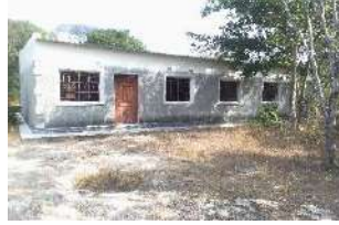
Staff house under construction
