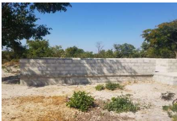
Incomplete Staff House
