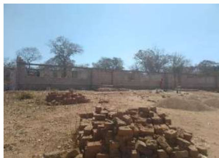
Incomplete 1x3 Classroom Block at Chisuku Community School
