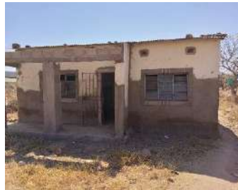
Incomplete staff house
