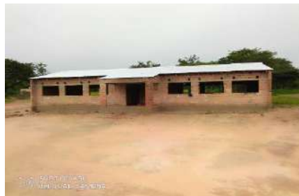
Incomplete classroom block
