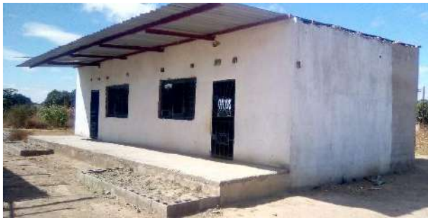
Stalled construction of a classroom
