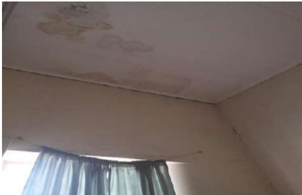
Leaking roof
