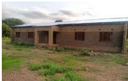
Incomplete Classroom Block at Kapata Community School
