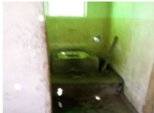
Toilet at Kamumanga Market
