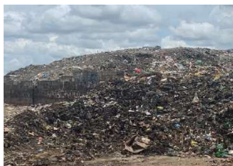
Waste overflowing the partial wall fence
