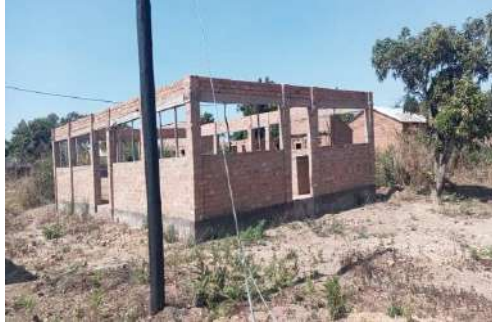
Incomplete market shelter at Kape
