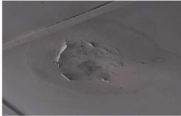
Leaking roof
