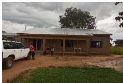
Stalled works at the maternity annex
