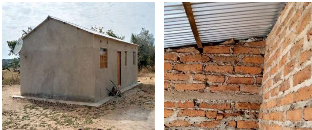
Incomplete staff house
