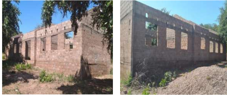
Incomplete 1x2 classroom block at Mundulundulu Community School
