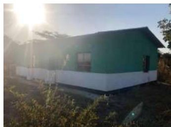
Staff house under construction
