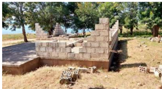
Incomplete Bar at Chipepo Guest House
