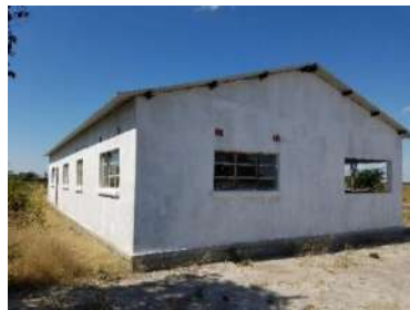
Incomplete structure for health post
