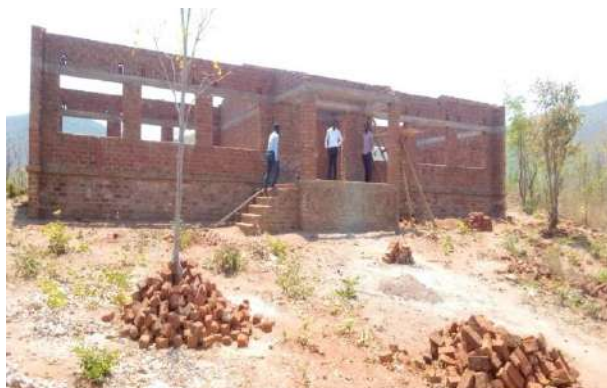
1x2 CRB under Construction
