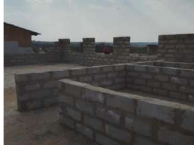
Incomplete 1x2 CRB at Sinungu Primary School
