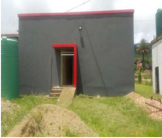
Incomplete Fire Station
