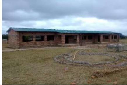
Incomplete 1x3 CRB at Changoma School
