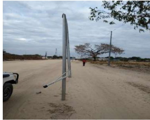
Vandalized Street Lights
