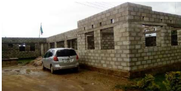
Mothers shelter at roof level
