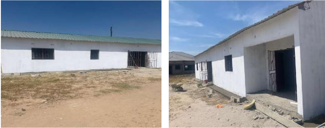
Incomplete at Mwalubemba clinic in Chinkuli Ward
