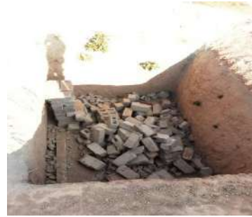
Demolished Septic Tank
