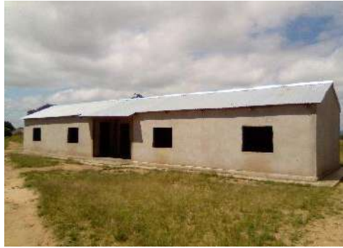
Incomplete staff house
