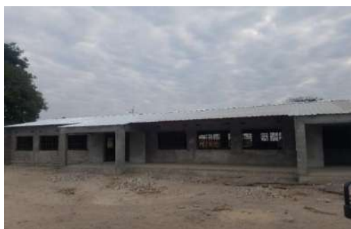
Incomplete 1x 3 CRB at Kashongo Primary School
