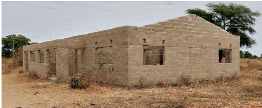
Incomplete staff house.
