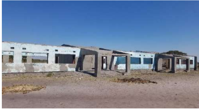
Incomplete 1x3 CRB at Mbumi Primary school
