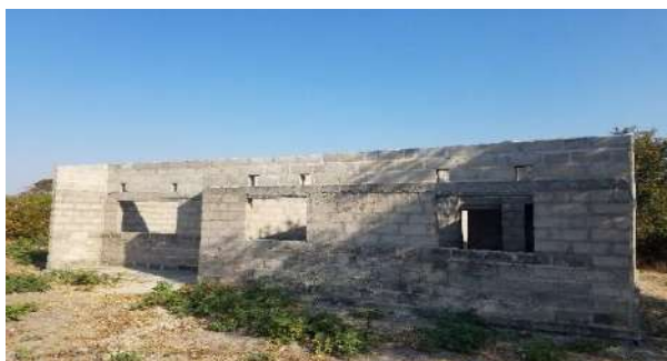
Incomplete staff House at Nalusheke
