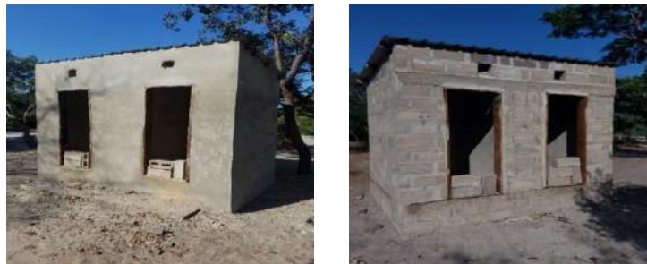
Incomplete construction of VIP toilets
