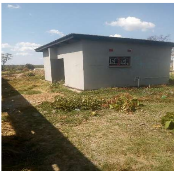
Completed ablution block
