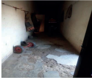
Corridor inside fire station
