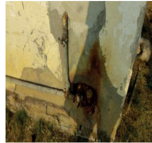
Leaking pipes
