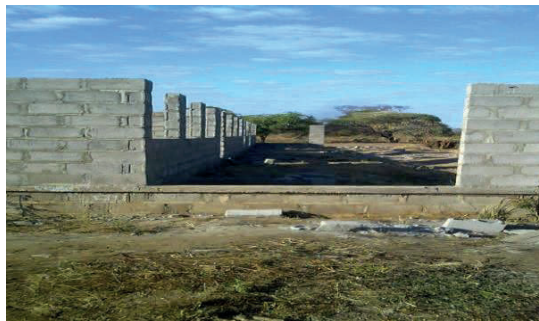
Unfinished construction of a 1 x 3 Classroom block
