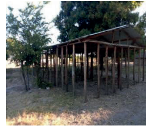
Uncompleted 6 th house
