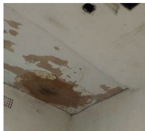
Leaking roof
