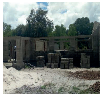
Incomplete classroom block
