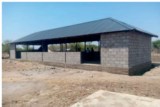
Incomplete market shelter
