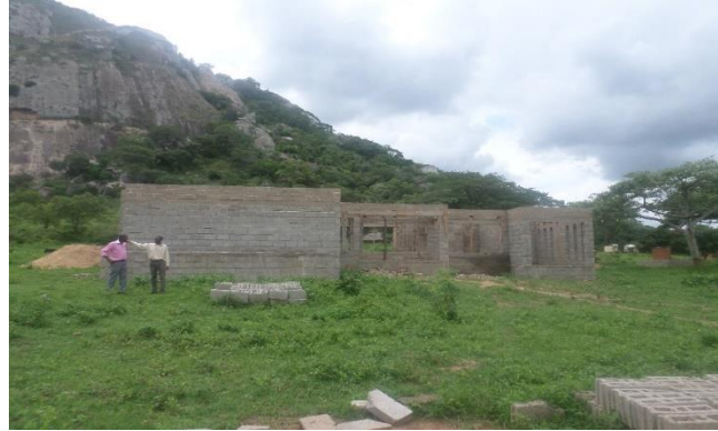
Chieftainess Nyanje's Palace at wall plate level
