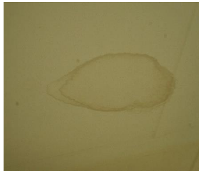
Leaking Roof
