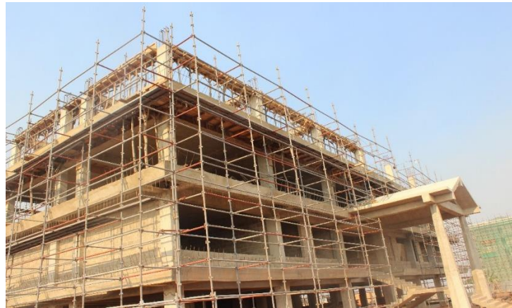
(4) Storey Office Block for the Provincial Administration under construction
