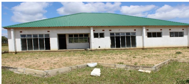
Post Office under construction in Mafinga
