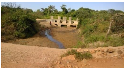
Construction of the culverts completed
