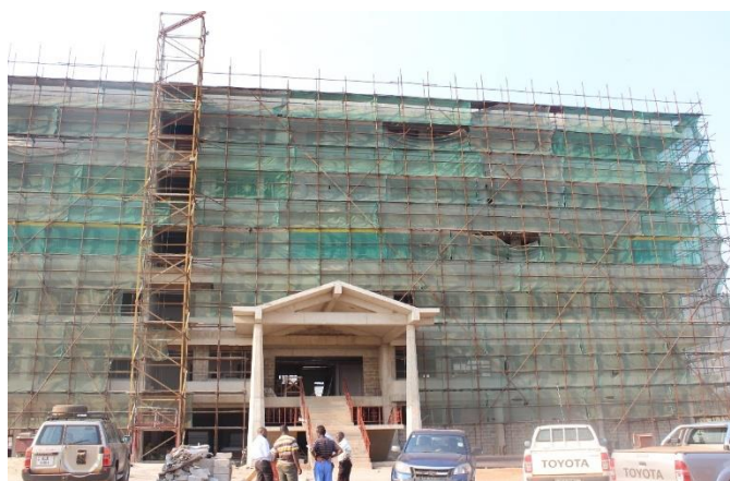
Six (6) Storey Office Block for the Provincial Administration under construction
