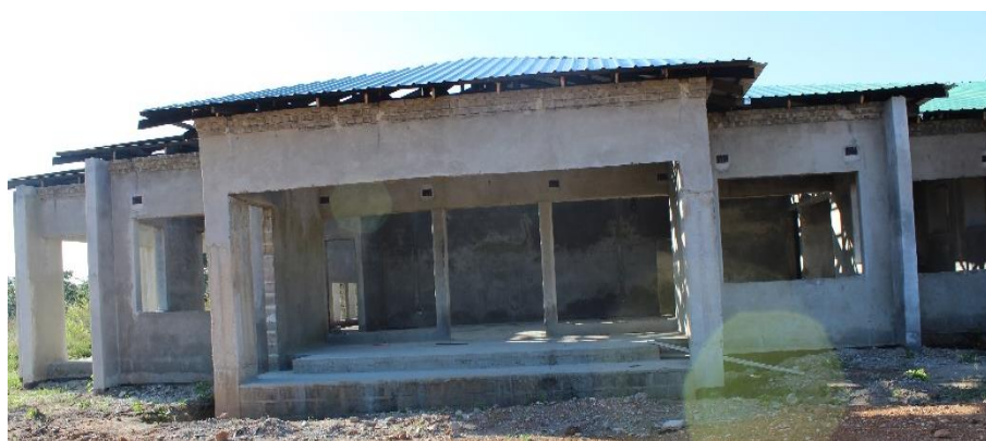
Post Office under construction in Shiwang'andu
