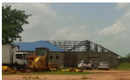
Partially completed office block
