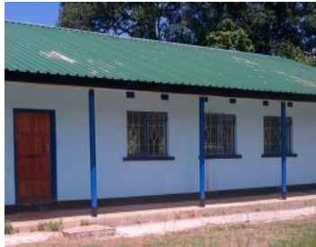
Corroding roof
