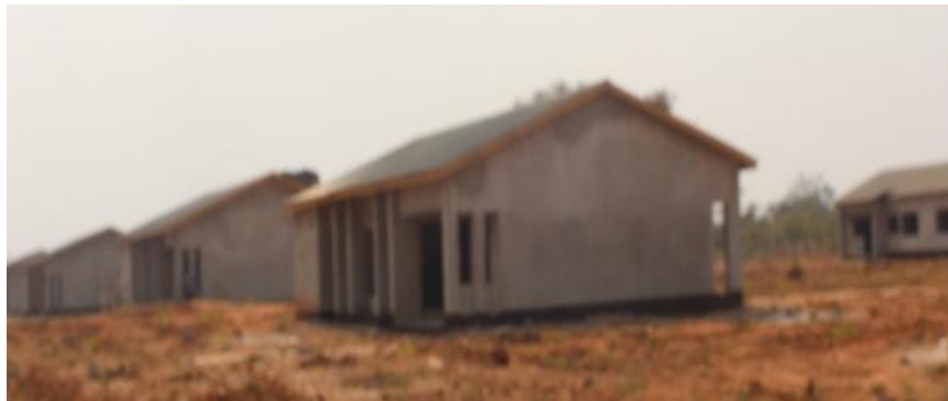
Part of twenty eight (28) houses at roof level
