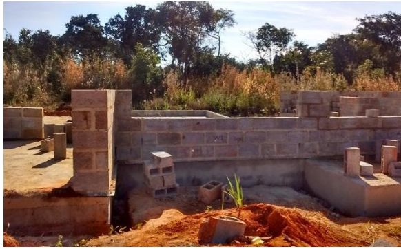
Chief Kalilele’s Palace under construction
