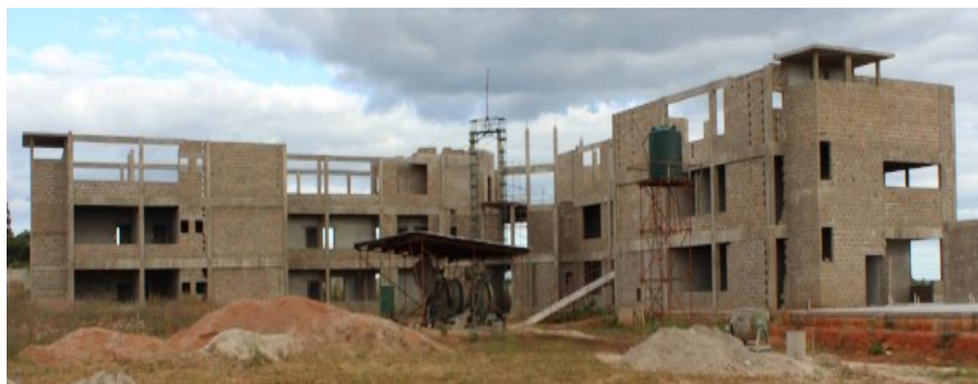
Civic Centre at wall plate level
