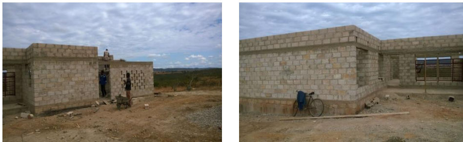
Construction at roof level
