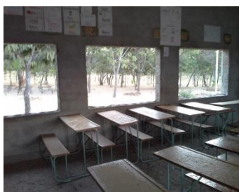
Inside one unfinished classrooms
