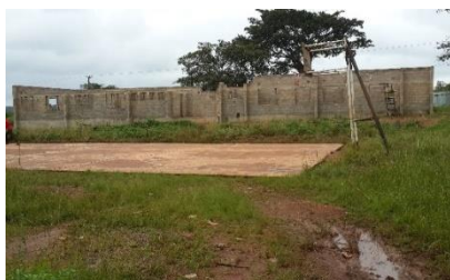
Front view of the Structure
