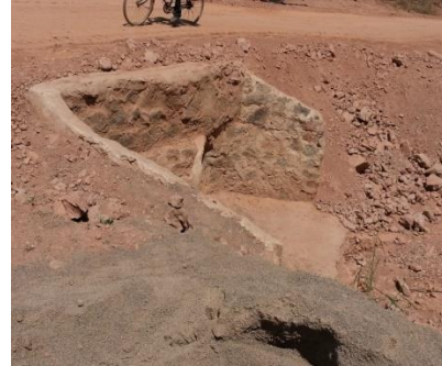
Outlet of the culvert
