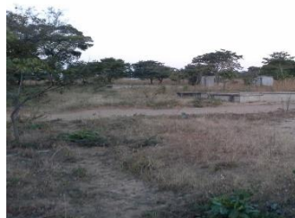
Abandoned staff houses at slab level
