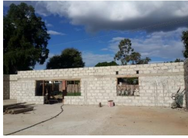
Structure at wall plate level
