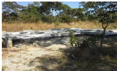
One of the houses at slab level
