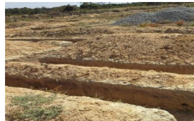
Excavations for the Administration block
