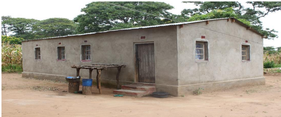
A rehabilitated staff house at Chimtengo Basic School with external walls not painted
