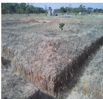
Excavations for the Assembly Hall 1 x 3 classroom block at gable level
