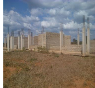
Two-storey lecture rooms at column level
