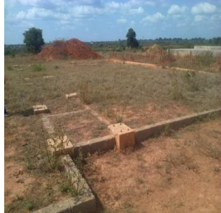
Lecture theatre at substructure level
