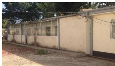
Front view of annex – 01/04/2014
