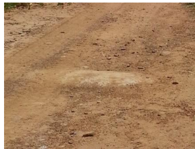
Exposed pipe culvert at 9.8km
