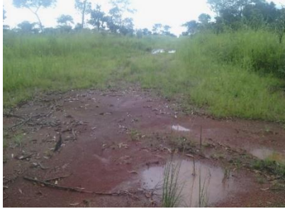
A stretch only bush cleared and light grading done
