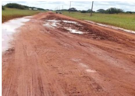
Water ponding at 8km and 20.3km respectively.
