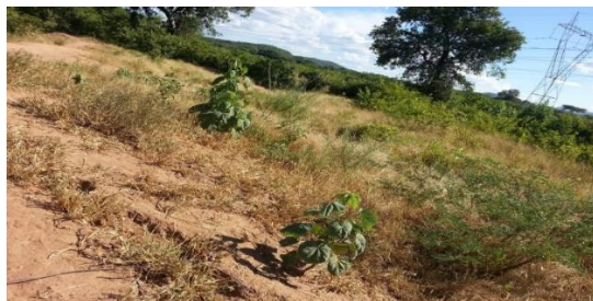
Uncleared shrubs in the spill way
