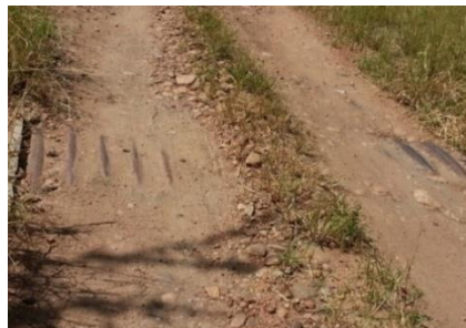
Exposed old culvert at 24.0km
