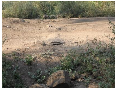
Broken down culvert not replaced at chainage 15.4km and road surface washed away at chainage 16.4 km
