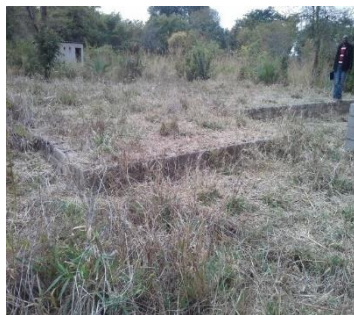
Classroom block at sub structure level
