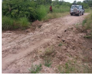
Section of road requiring culvert at 3.3km Section of road requiring culvert at 10.3km
