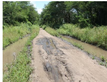
Broken down culvert not replaced at chainage 15.4km and road surface washed away at chainage 16.4 km
