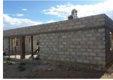
Structure at wall plate level
