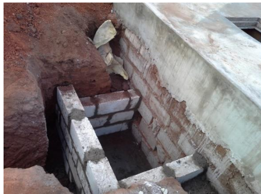
Soaker way under construction
