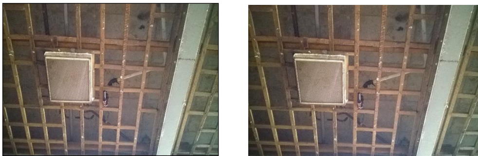
Old Waste Water Lines
