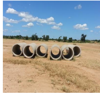
Culverts not installed at 10.5km
