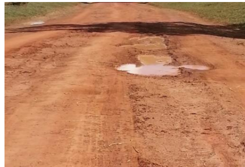
Water ponding at 8km and 20.3km respectively.
