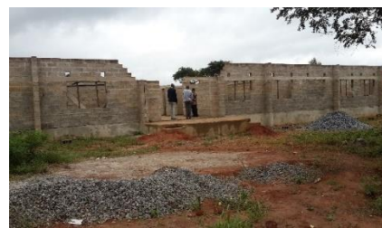
Rear view of the structure
