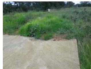
Incomplete Slab for Boys Hostel
