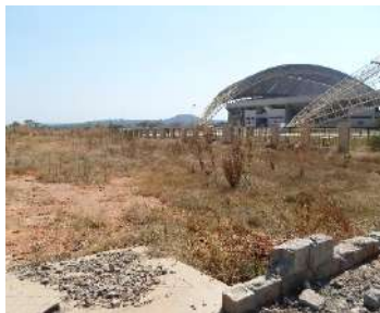
Part of the worked on car park
