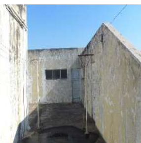
Roof top of the Chancery
