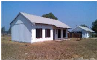
Prefabricated house under construction
