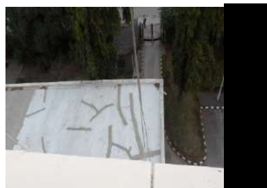
Part of the mended roof at the Chancery
