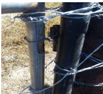
Gate detached at the hinge of one end
