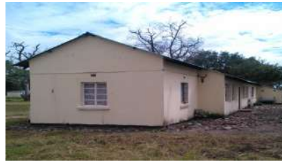
The roof without fascia board
