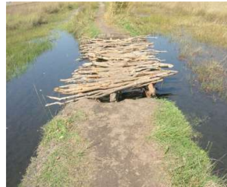
Parts of the eroded embankment with temporal bridge constructed by the community.
