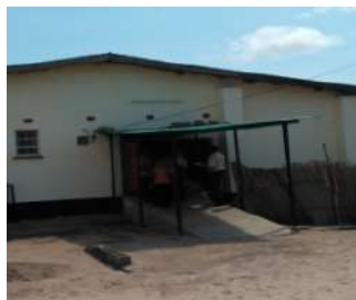
The flat roofed ramp
