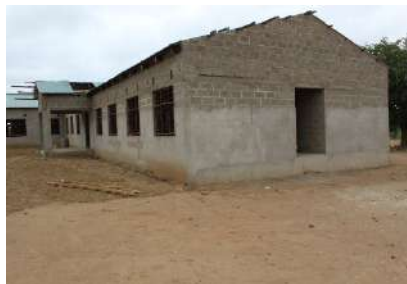
An incomplete Vubwi DC's office block
