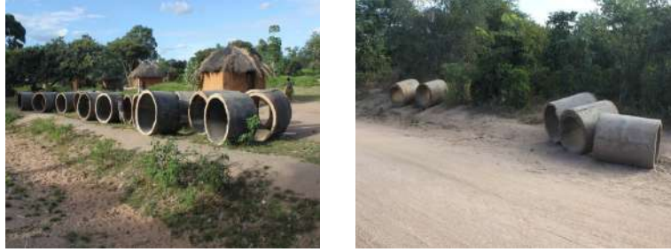
Culverts meant for drainage works along the Nyati – Simambumbu Road
