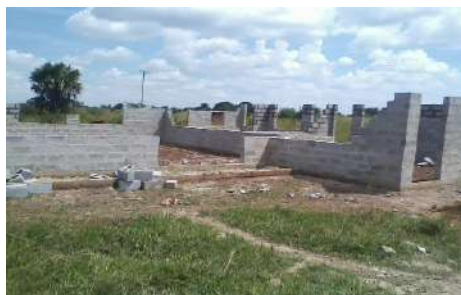
Community Hall under construction in Shibuyunji District
