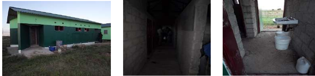
The Ablution Block with the remaining works
