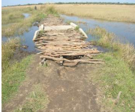
Parts of the eroded embankment with temporal bridge constructed by the community.
