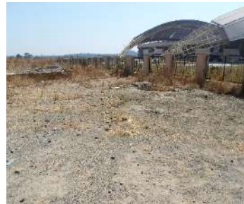
Worked on car park
