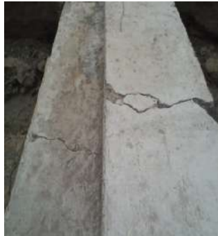
Original Crack
