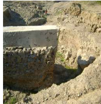
Gully at end of head wall
