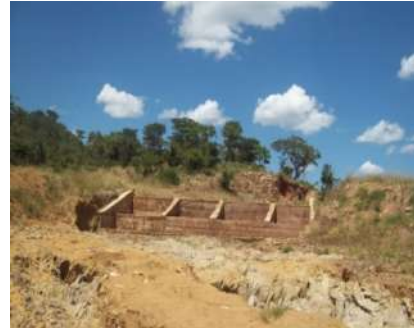
Opening on the wall of Konkola dam
