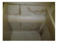
Damaged ceiling due to leakages
