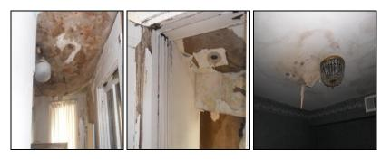
Damaged Ceiling Boards in the interior of the house
