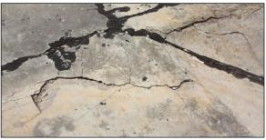
Cracks on concrete walk way
