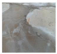
Cracks on the rehabilitated Air craft washer
