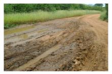
Water ponding and Wheel ruts formed at 6.9km
