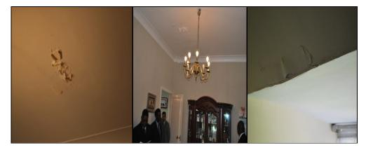
Damaged ceilings at the Residence due to leakages
