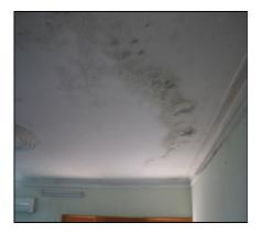
Rain damaged walls and ceiling
