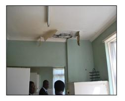
Damaged leaking ceiling
