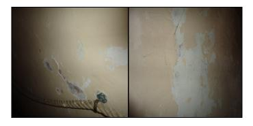
Paint peeling off the basement wall s
