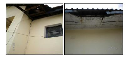
Cracked wall and damaged roof at 6 Lundula Avenue
