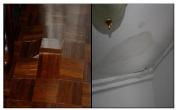
Wooden floor tiles coming off Damaged ceiling board
