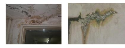
Part of concrete ceiling showing leakages
