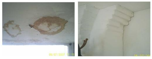
Peeling paint on the wooden walls and cracks between wooden walls and pillars
