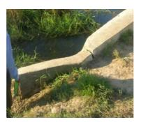
A crack on the culvert head
