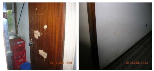
Broken door and wall with patches that needs replacement and maintenance
