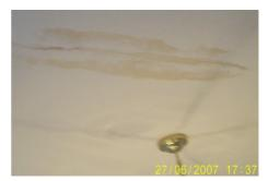
Peeling paint due to leaking roof
