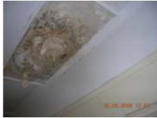
Damaged ceiling as a result of the leaking roof
