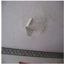
Damaged ceiling and peeling off paint due to defects in the roof
