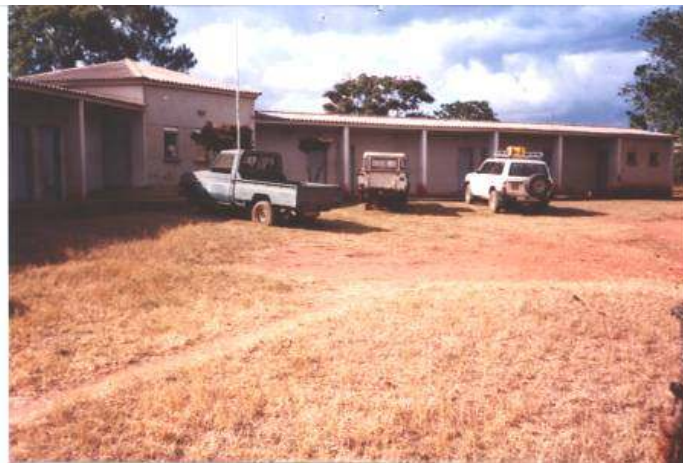
Disused Hostel Block – Chipata (Front View).
