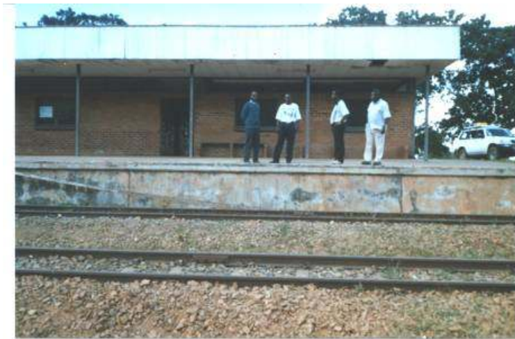
Constructed Railway Station in Malawi
