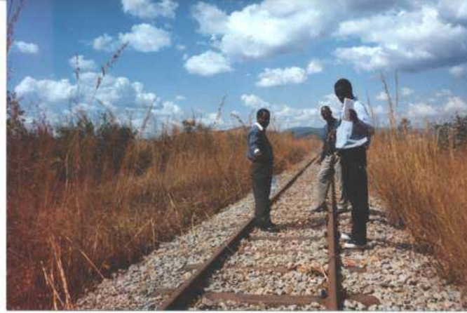
30kg rail line constructed on class ‘A’ steel sleepers (Zambia).
