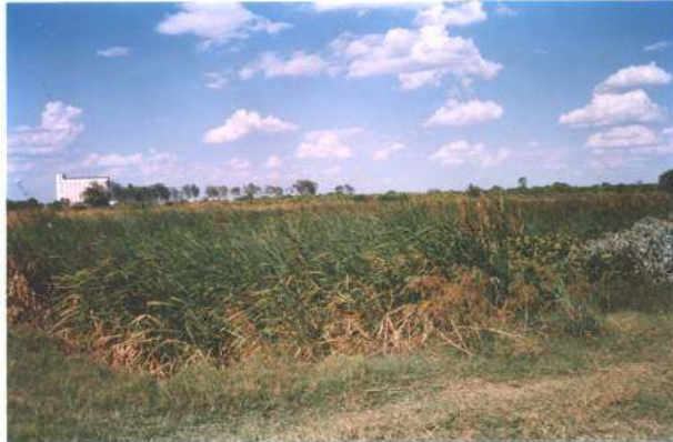
Overgrown vegetation – Ngungu sewer ponds
