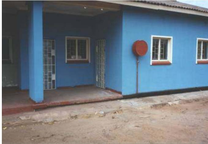
Front view of rehabilitated Livingstone TRC office
