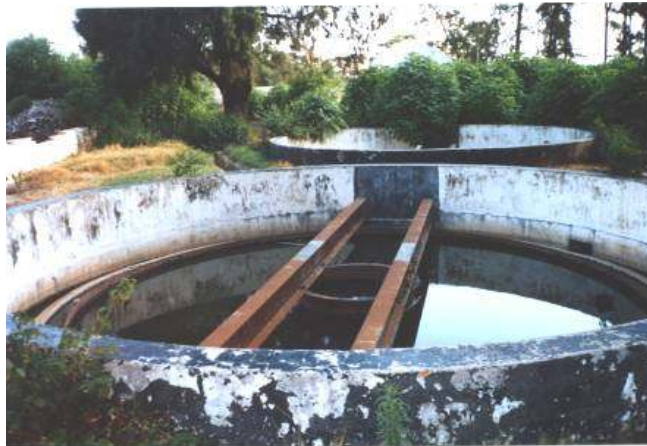
Defunct treatment Plant
