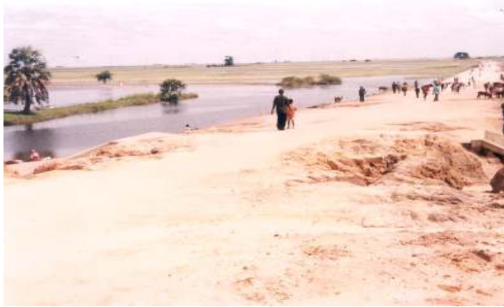
The beginning of the Mongu-Kalabo road at Mulamba Harbour
