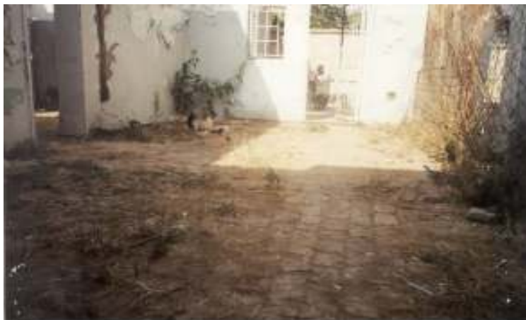
Permanent Secretary's official residence under renovation – Front view
