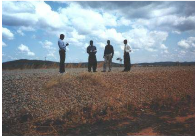
Ballast material left on site which follows formation of rail track.
