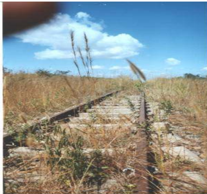
40kg rail-line constructed on concrete sleepers (Malawi).
