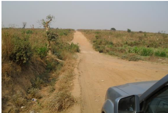
Road section at chainage 1.6 to 2.6
