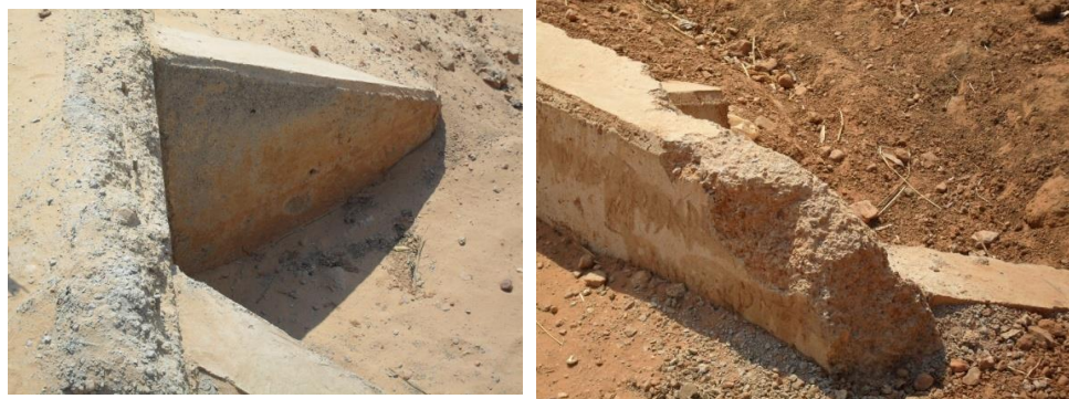
Broken Headwalls
