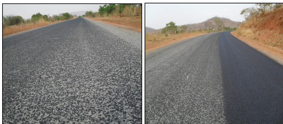
Worn out surface due to non holding of Second seal (l) Fog spray (r)
