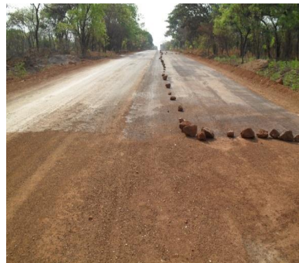
Primed road used for traffic
