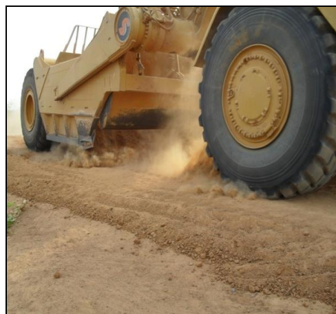
A scraper applying soil on the road
