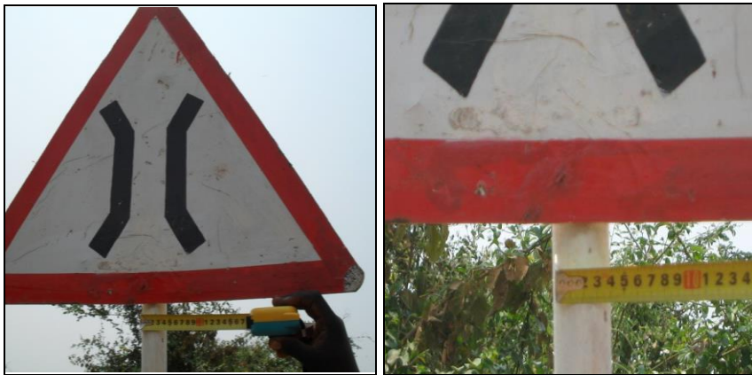
Road sign on a thin post (4.5cm external diameter) at KM 48.7
