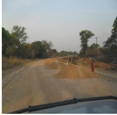
Heaps of gravel fill not spread
