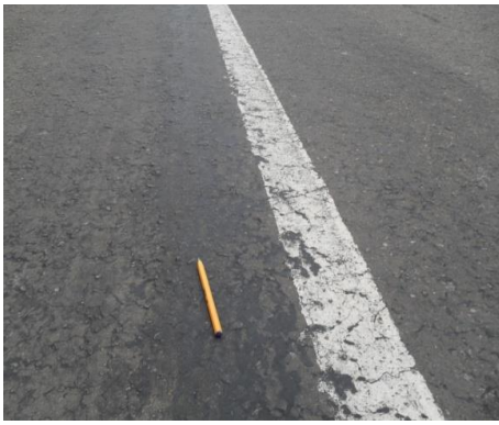
Road marking fading due to bleeding (l) and Signs of bleeding Ch 42.6km (r)
