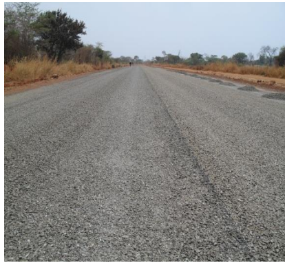
Surface dressing 1 st layer
