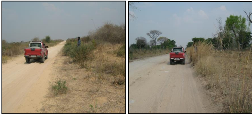
Tall grass and evidence of shrubs close to the road
