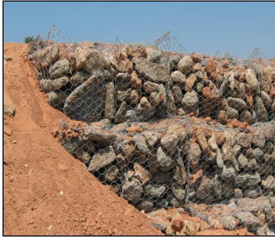
Loosely packed stones in gabion baskets
