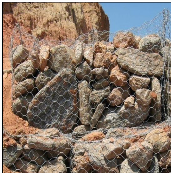
Oversize stones used in gabion baskets
