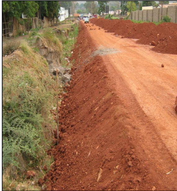
Obote road certified for 150mm, 3% cement stabilized base but not done
