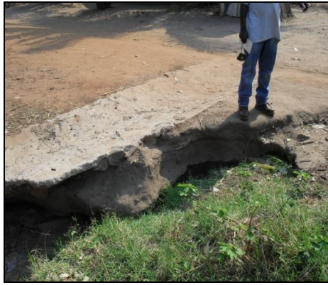
The drift and the wash out at 0.5 km
