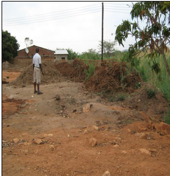
Part of the cut to spoil material
