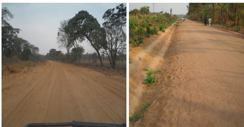
Road Bed with dust (l) and Road bed formed without gravel fill(r)
