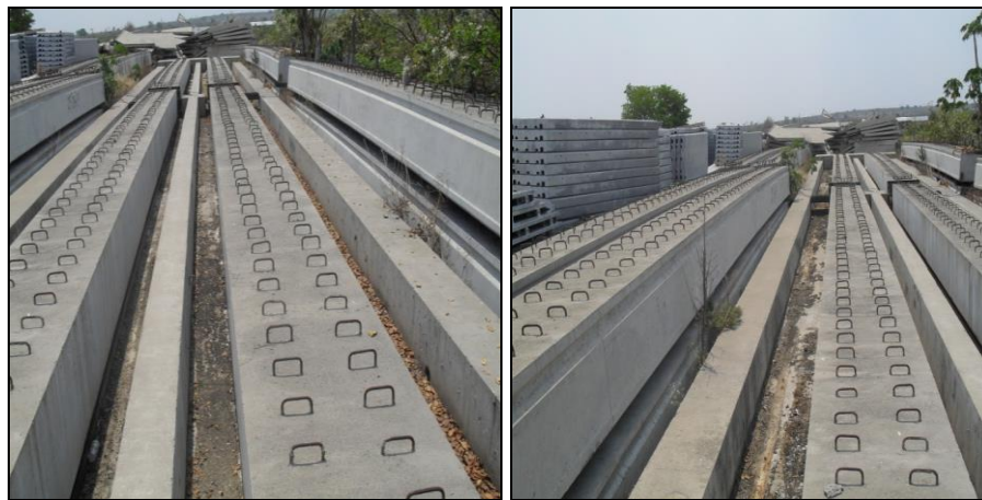
Pre cast-concrete beams meant for construction of bridges along Mongu - Kalabo flood plains
