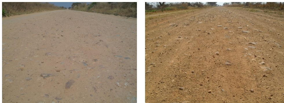
Stones on the Gravel Material
