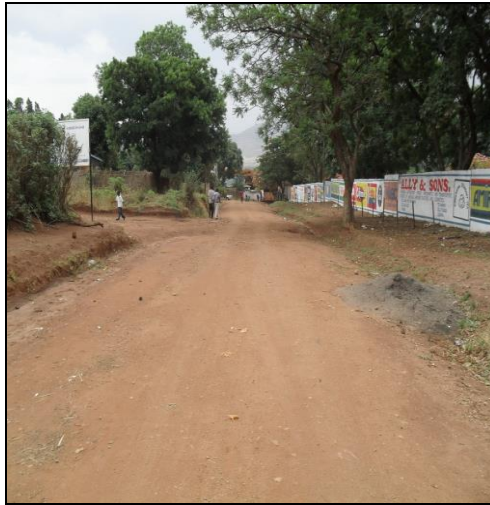
Existing township road earmarked for clearing and grubbing
