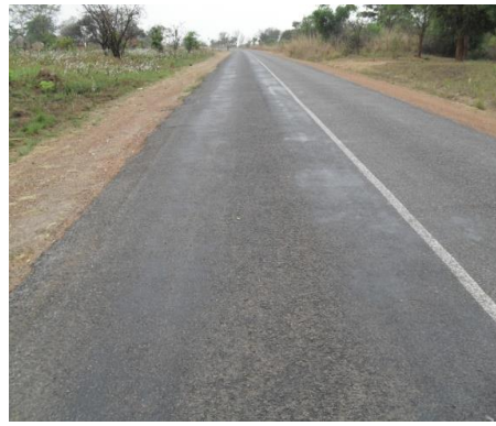
Road marking fading due to bleeding (l) and Signs of bleeding Ch 42.6km (r)
