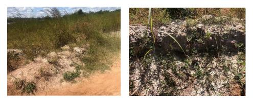
Sand bags on the eroded dam embankment
