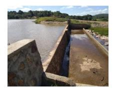
Spillway and embankment requiring raising
