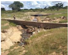
Layed sacks and gabion baskets on training wall The eroded spillway requiring repairs
