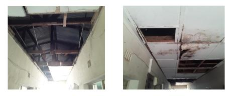
Traces and Ceiling Boards Damaged by Termites
