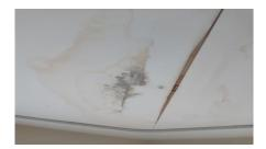
Stained ceiling due leaking roof
