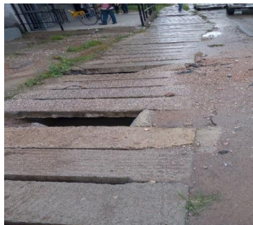
Damaged Drainage Concrete Covers along Chozi Road at Northmead Market
