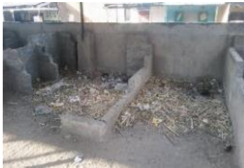
Uncompleted Market Stands
