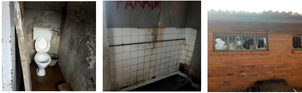
Toilets and Office block at the Cleansing Depot
