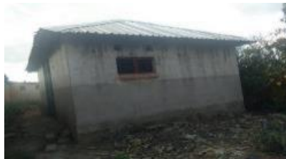
Uncompleted Ablution Block.
