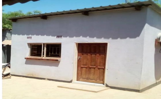
Office structure constructed on a private property
