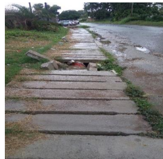
Damaged Drainage Concrete Covers along Chozi Road at Northmead Market
