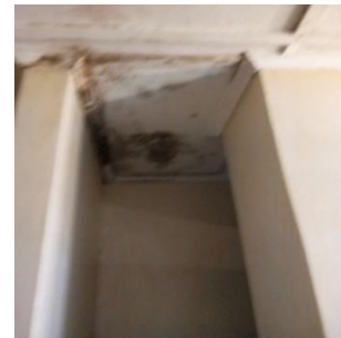
leaking ceiling
