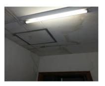
Stained ceiling and Visible Cracks
