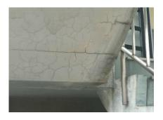
Cracks under the Third Floor Stairway
