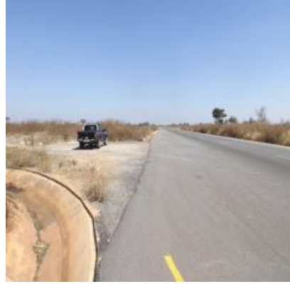
Bell mouths not surfaced at the road edge within MFEZs
