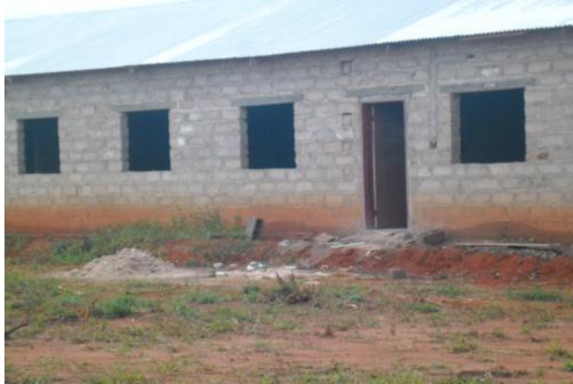
Construction works at the camp site for Mpika – Nabwalya Lot 1
