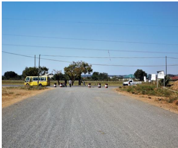
Utility cable with low clearance
