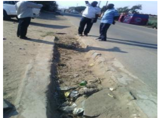
Uncompleted works with drainage which had no direction of discharge flow (Lot 7 A3)
