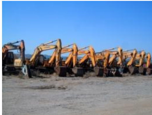
Equipment parked due to work stoppage
