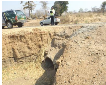
Culvert without headwalls along the Chipata - Mfuwe Road
