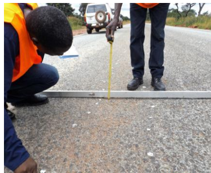
Surface Irregularities observed using a 3 m straight edge
