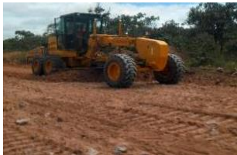
Clearing and Grubbing works along Mpika – Nabwalya Lot 1
