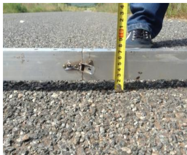
Surface Irregularity on the road
