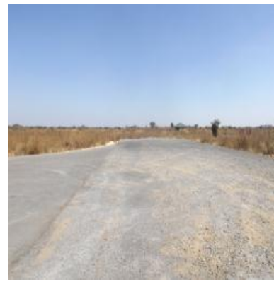
Bell mouths not surfaced at the road edge within MFEZs
