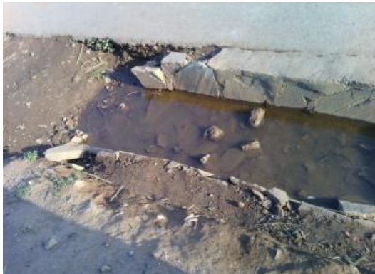
Uncompleted works with drainage which had no direction of discharge flow (Lot 7 A3)
