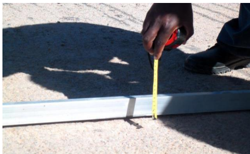
Visual inspection of rutting or surface regularity
