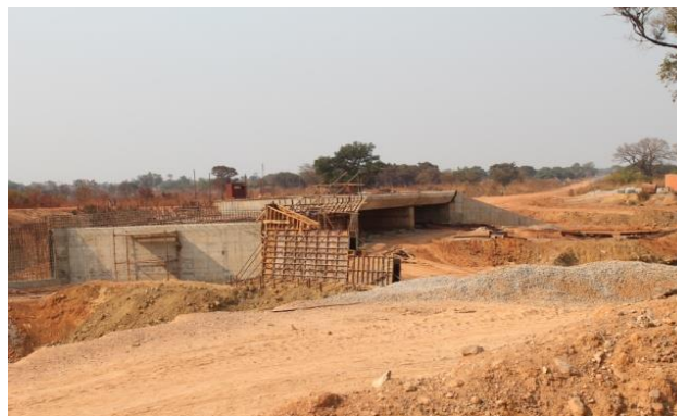
Bridge still under construction
