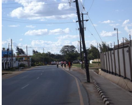
Electricity poles less than 1 metre from the edge of the carriage way
