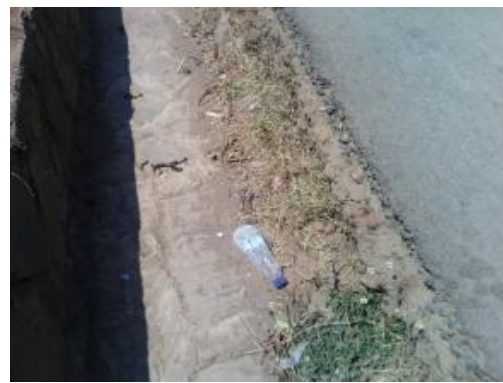
Unpitched walls of drainage (Lot 7 A4)
