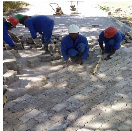
RDA staff manually laying pavers at Mansa General Hospital
