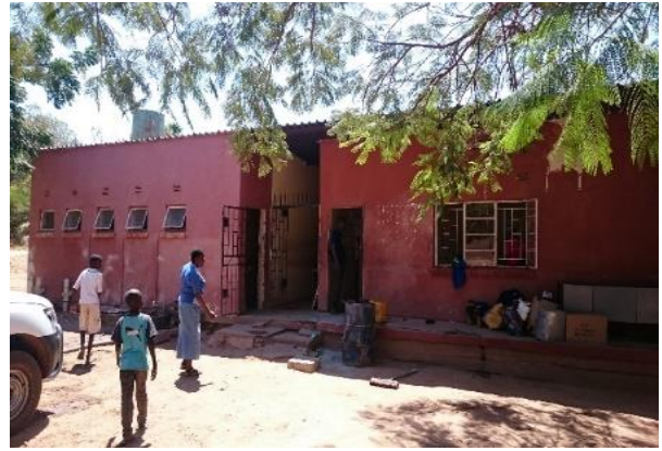
Front side of the ablution block housing a fire brigade office
