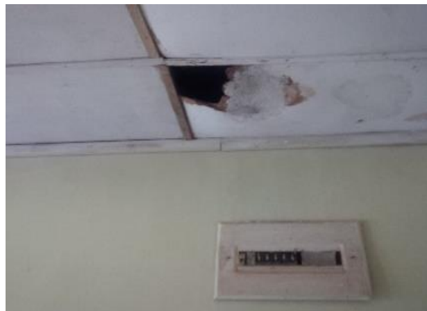
Peeled tiles and fallen ceiling in the Guest House
