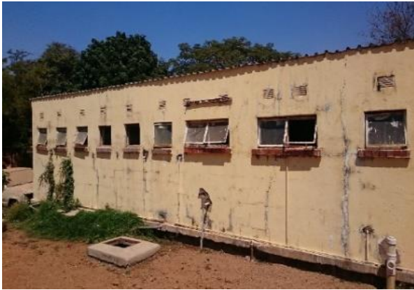
Rear side of the ablution block housing a fire brigade office
